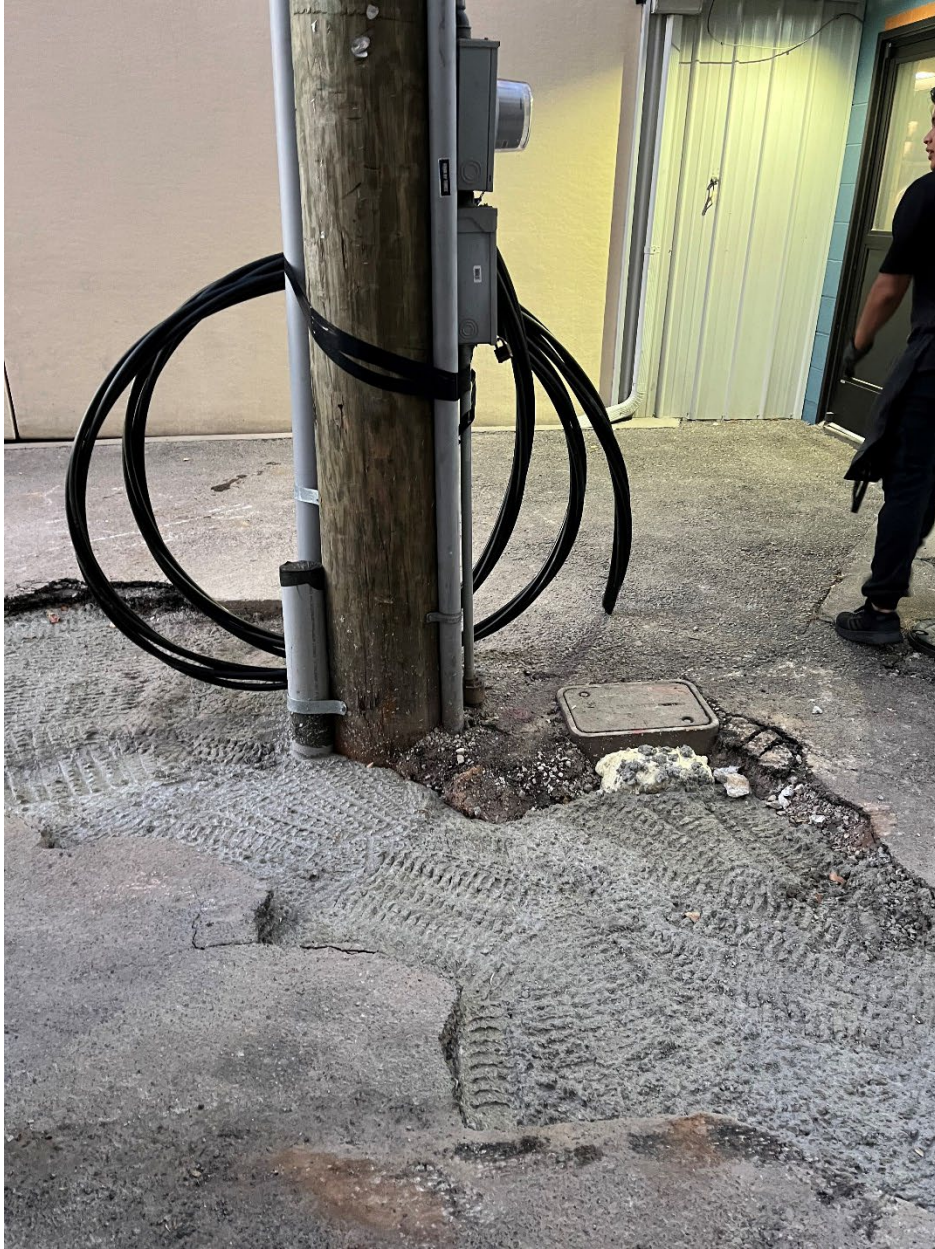
Newly installed Duke power lines from 8/31/23
