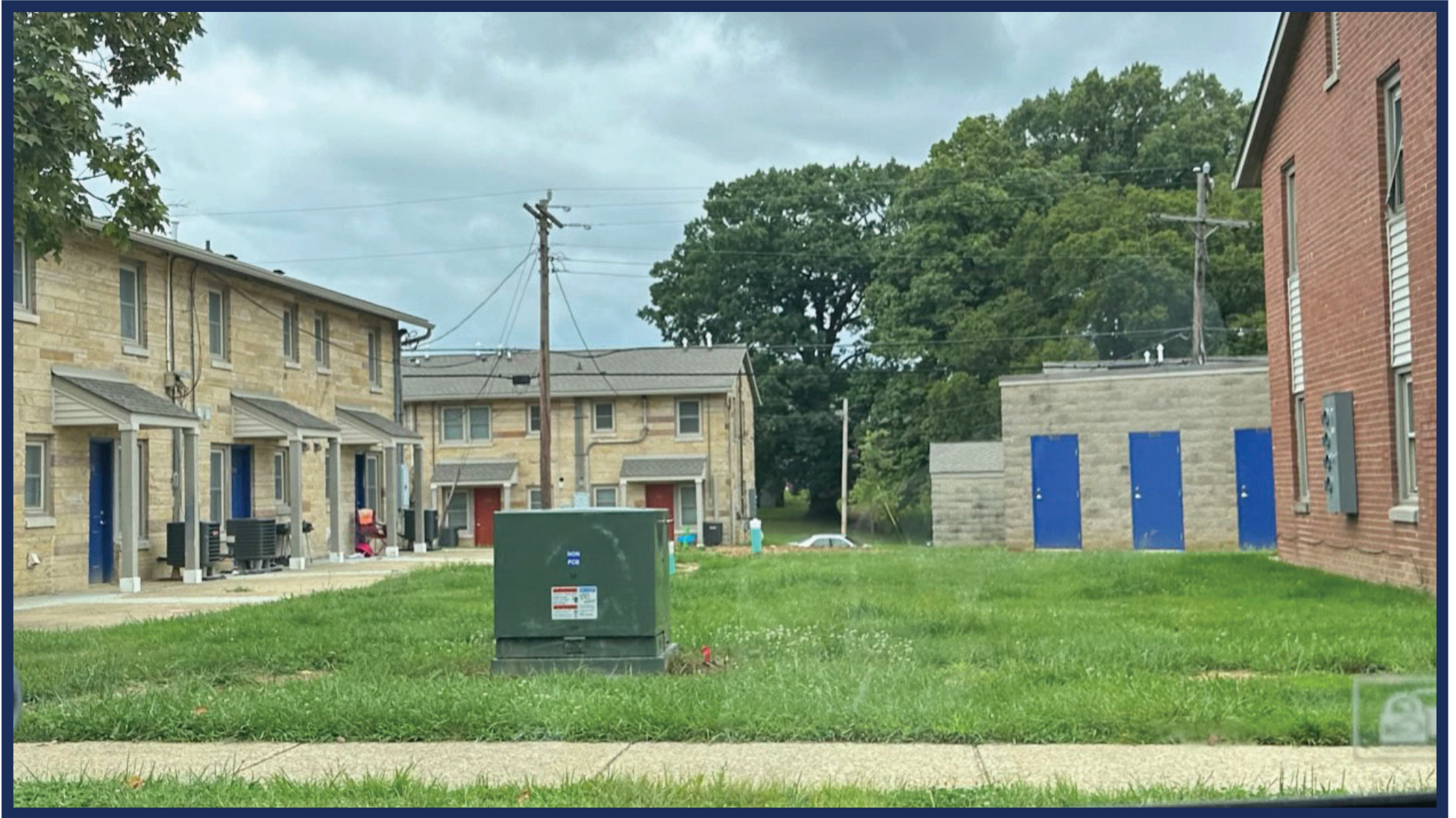
Crestmont Community (1007 N Summit St., Bloomington, IN) Photo 4 Site Visit September 5, 2023 12th street facing north
