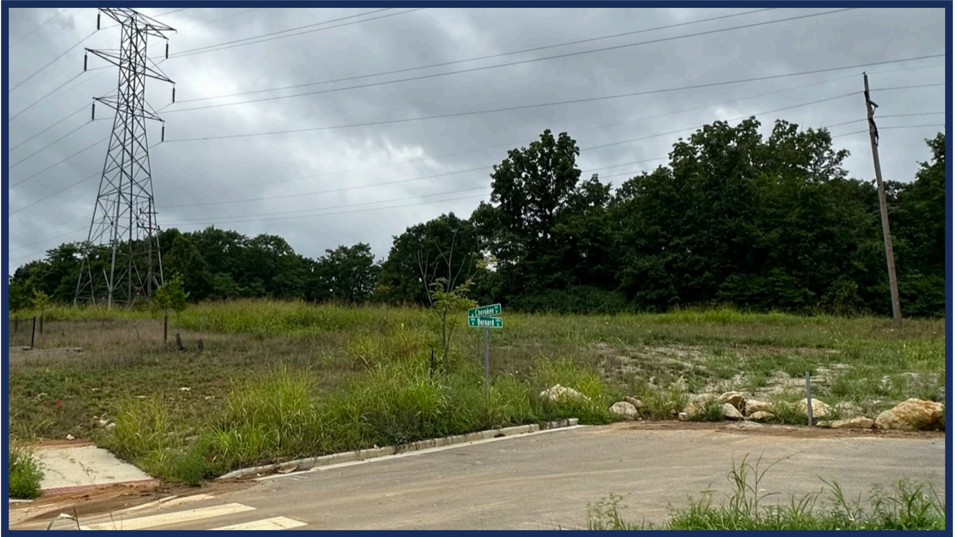
Osage Place, Habitat for Humanity, Bloomington, Monroe County, Indiana Photo 4 Site Visit September 5, 2023 Standing on the corner of S Bernard and Cherokee Drive facing northwest
