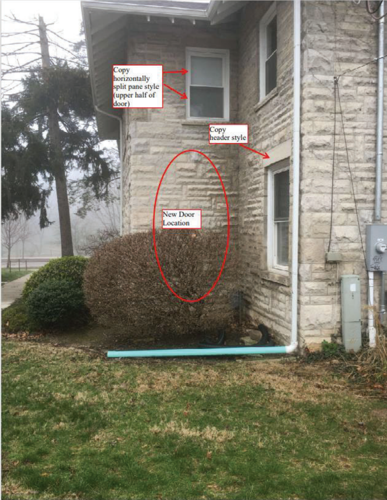
Figure 4 Design concept of Exit door
