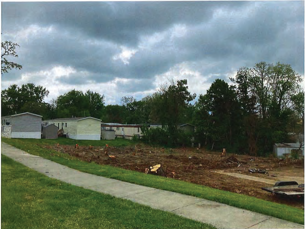
Photo 3: Earth disturbance, absence of erosion control measures, and trees removed on the northern side of 1450 N Willis Drive on 05/12/2023.
