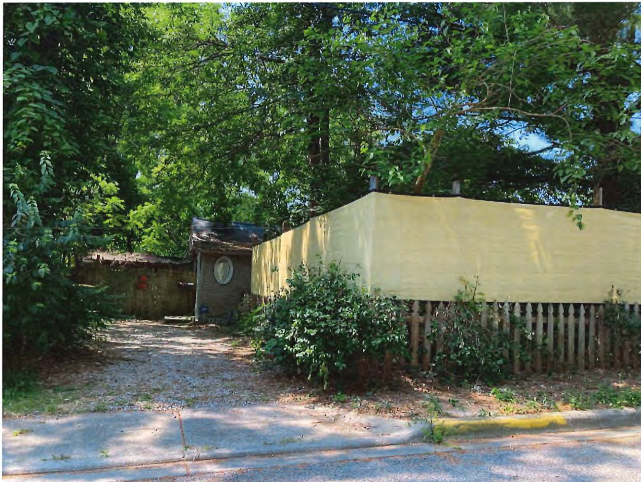
Photo 1: Fencing in excess of 4 feet in height forward of the front building wall at 1207 W Cottage Grove Ave on 06/08/2023.
