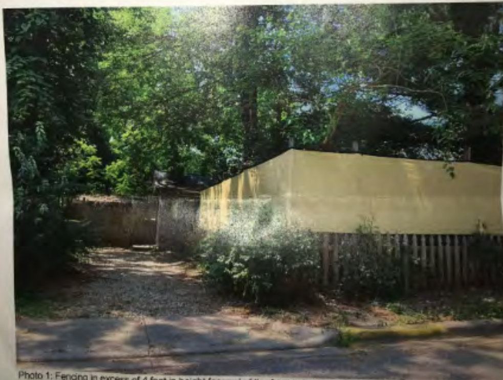
Photo 1: Fencing in excess of 4 feet in height forward of the front building wall at 1207 W Cottage Grove Ave on 06/08/2023.
