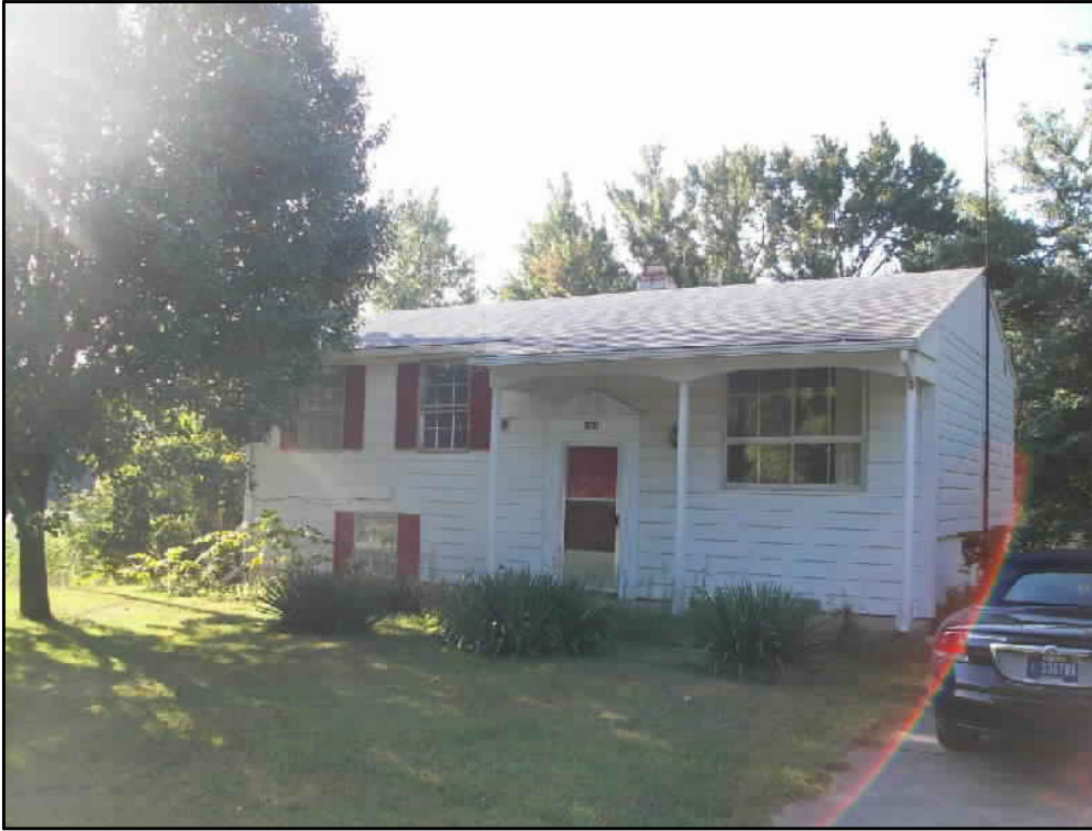
FRONT VIEW OF SUBJECT PROPERTY
