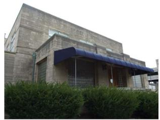
The layered cornices are corbelled with three belt courses and the coping is curved. Windows are large industrial metal windows which seem to have been modified from the original design.
