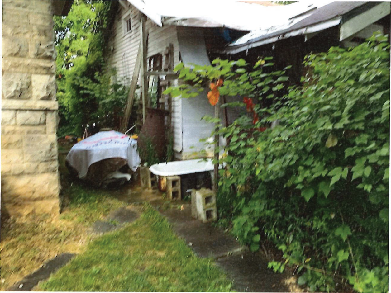
Photo 2: Storage of materials on the south side of 530 S. Washington Street.
