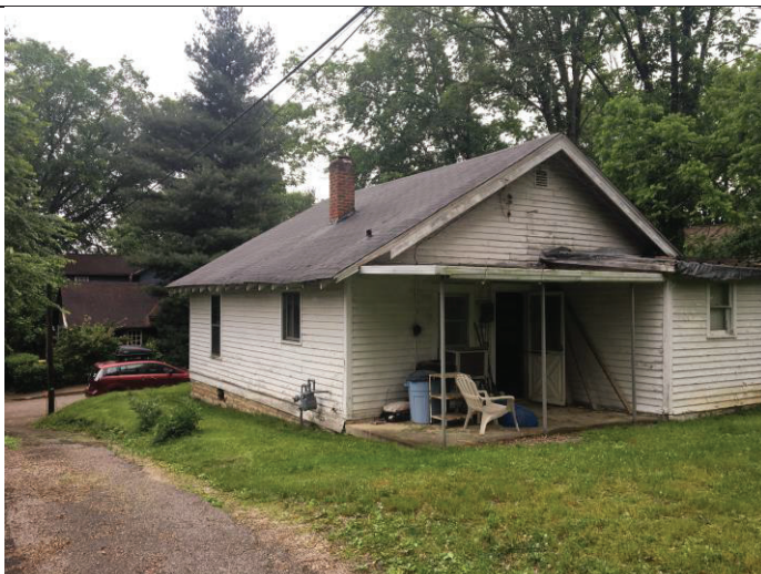
South Elevation, looking west along alley
