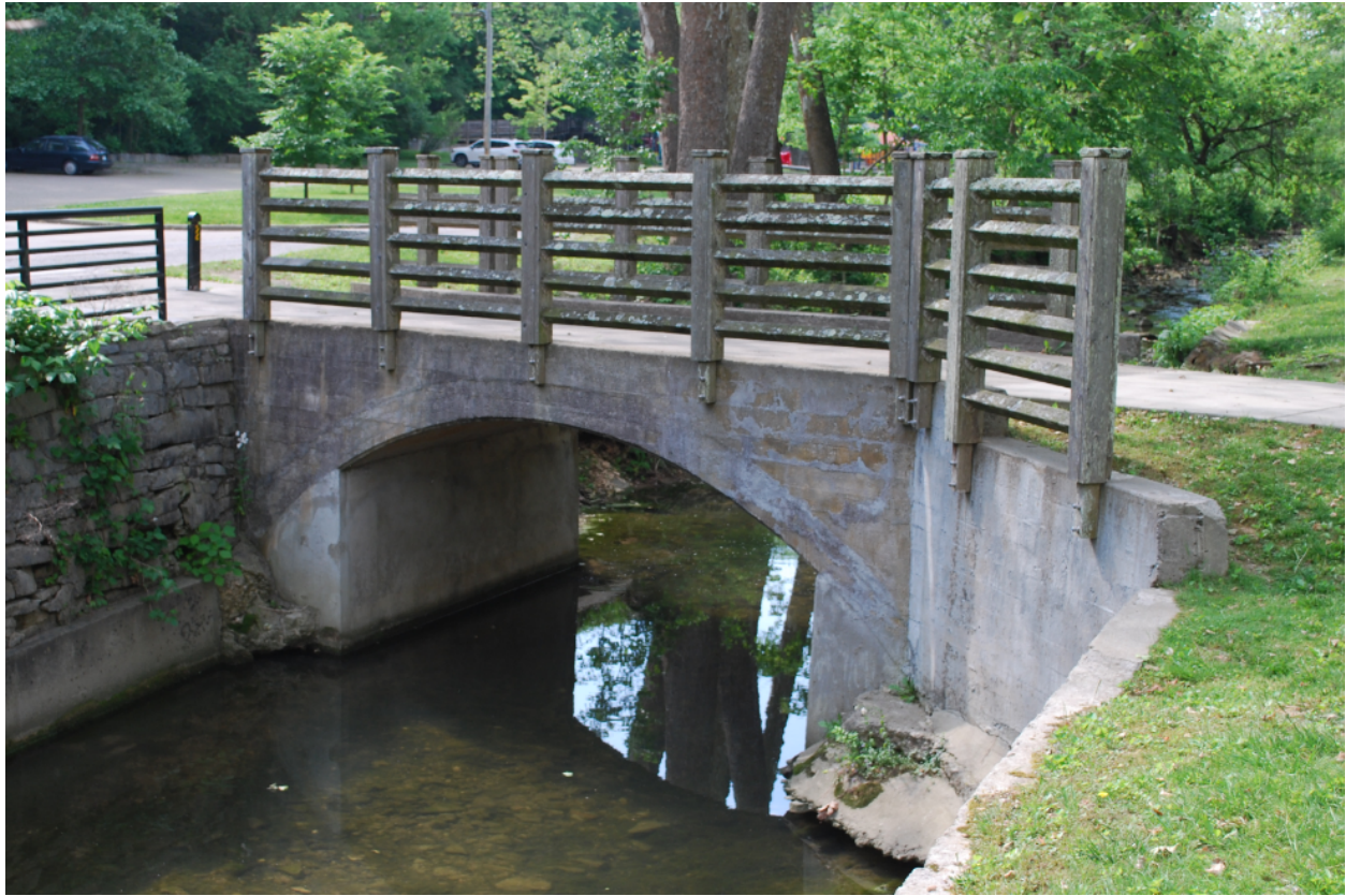
Image 8: Concrete Pedestrian Bridge, looking southwest
