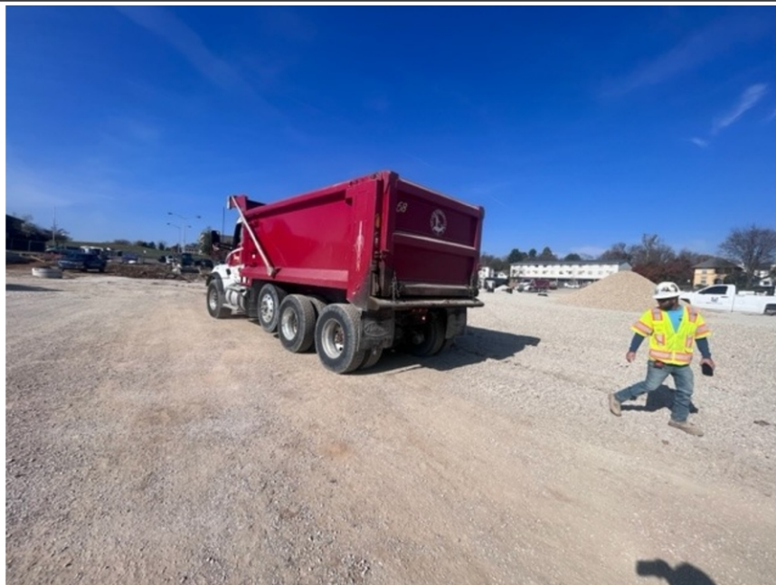
View of proofrolling on University street.
