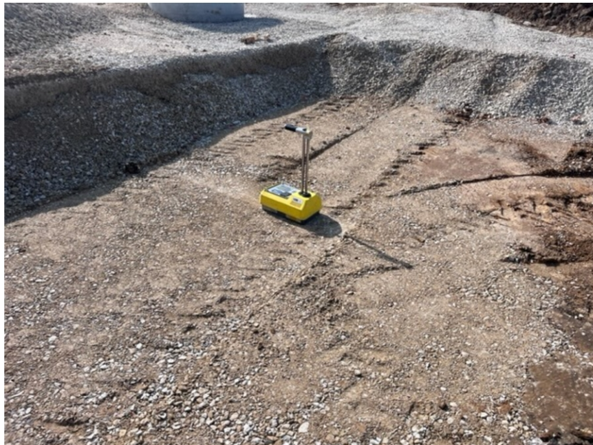
View of compaction testing.
