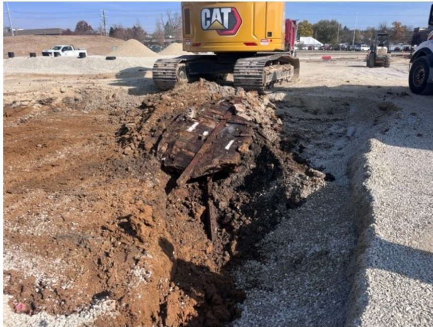
View of trash and debris removed from undercut #2.
