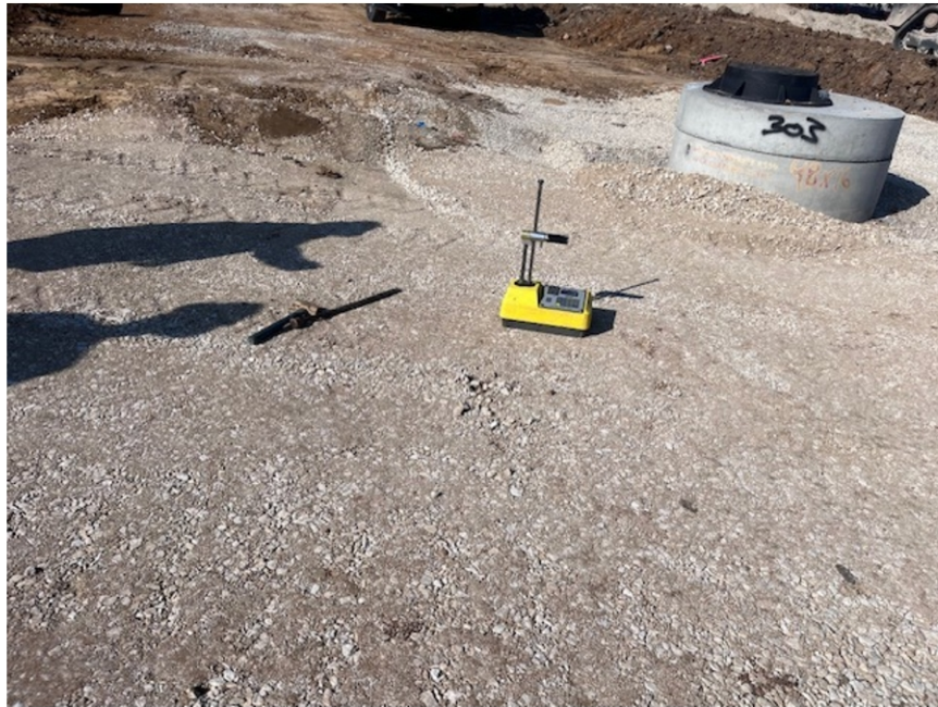
View of compaction testing.
