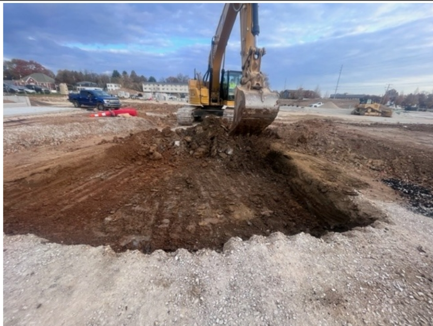
View of unsuitable soils being removed.
