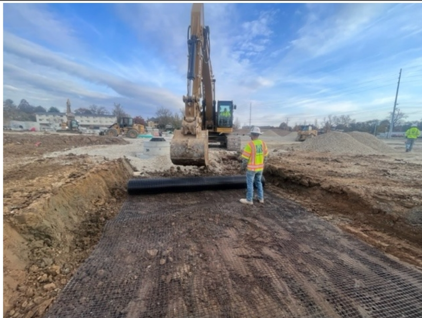
View of undercut and geogrid placement.
