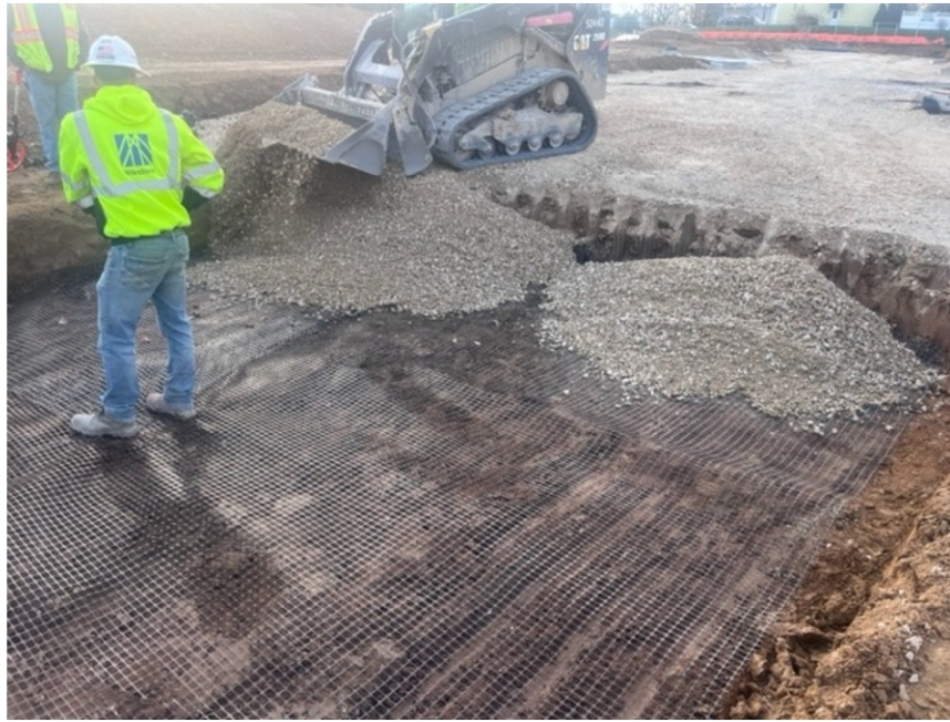
View of #53 stone being placed on the geogrid in 12 inch lifts.
