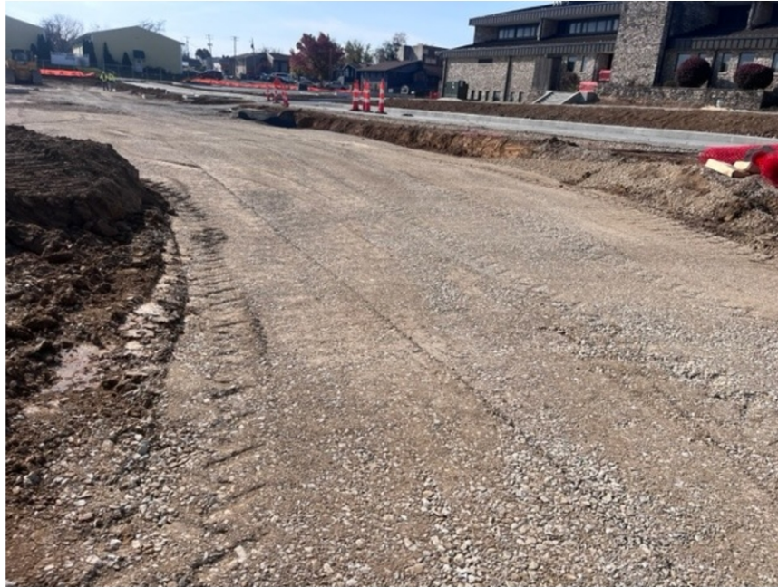
View of Undercut # 1 Completed.
