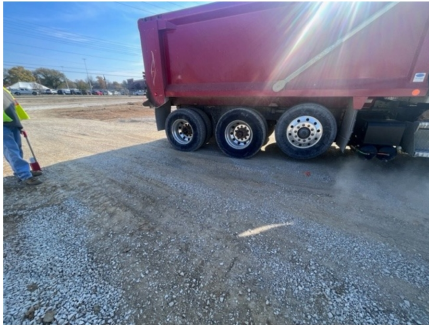
View of proofrolling on University street.
