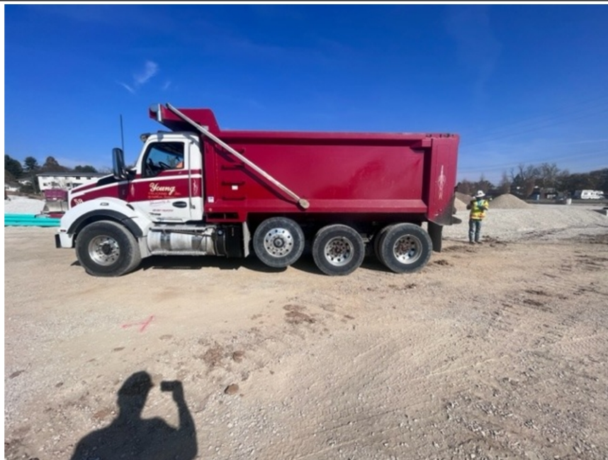
View of proofrolling on University street.
