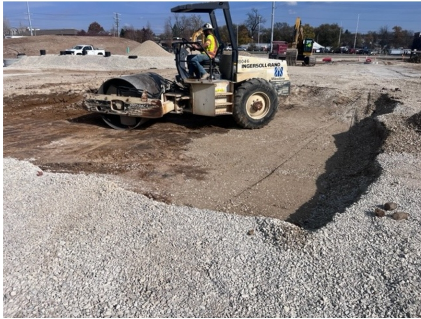
View of compaction of #53 stone after removing unsuitable soils.
