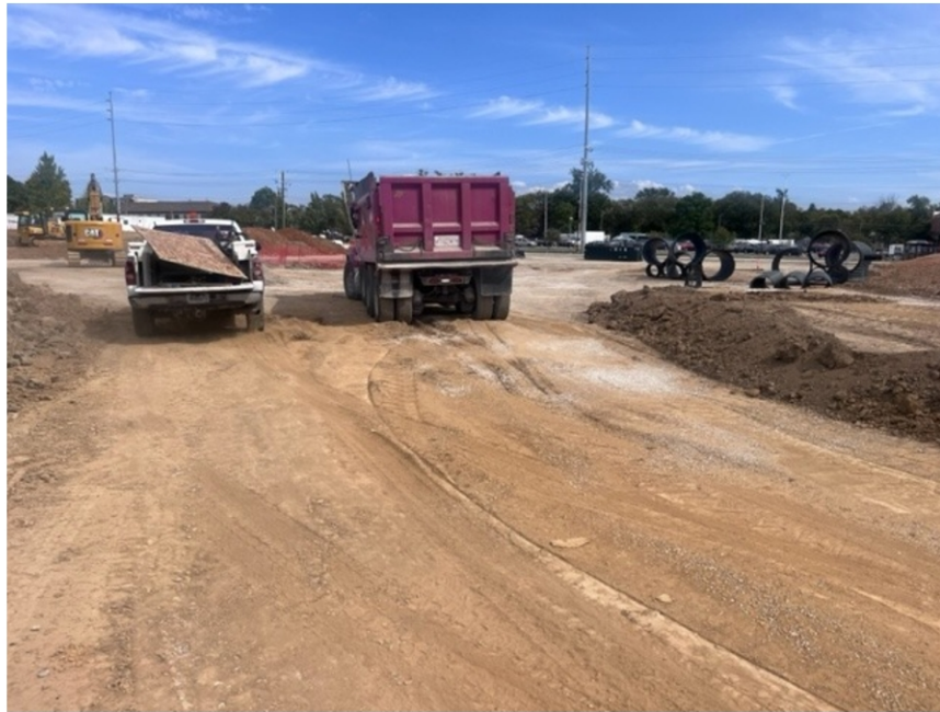
View of the Subgrade at the time of Proofrolling facing North.
