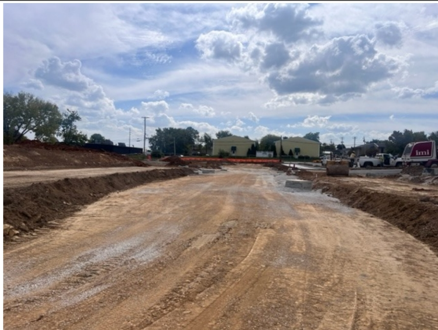
View of the Subgrade at the time of Proofrolling facing South.
