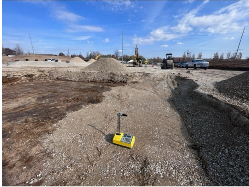
View of compaction testing.
