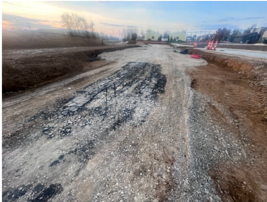
View of undercut location #1 prior to removal of unsuitable soils.
