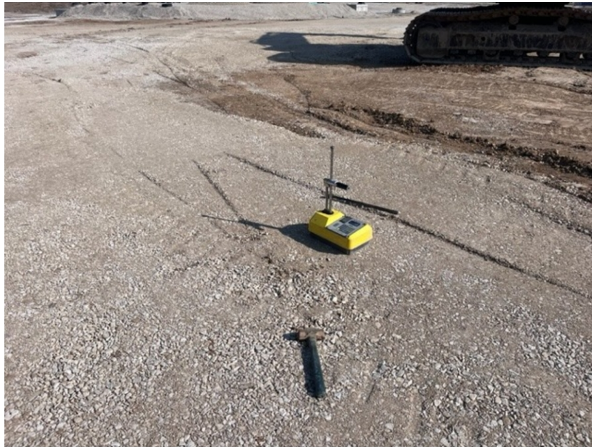
View of compaction testing.
