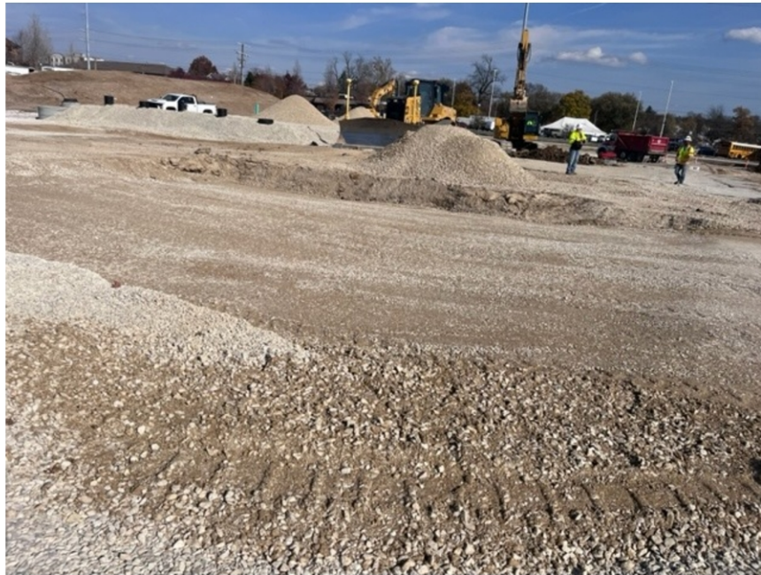
View of first lift of undercut location #2 after compaction.
