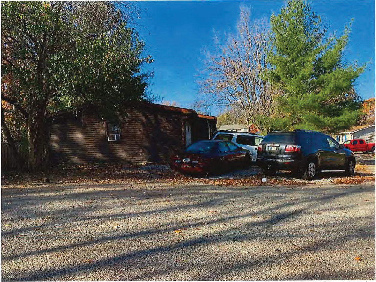
Photo 3: Driveway exceeding the allowed width on the northeast side of the property at 1205 W East Branch Drive on 11/09//2023.
