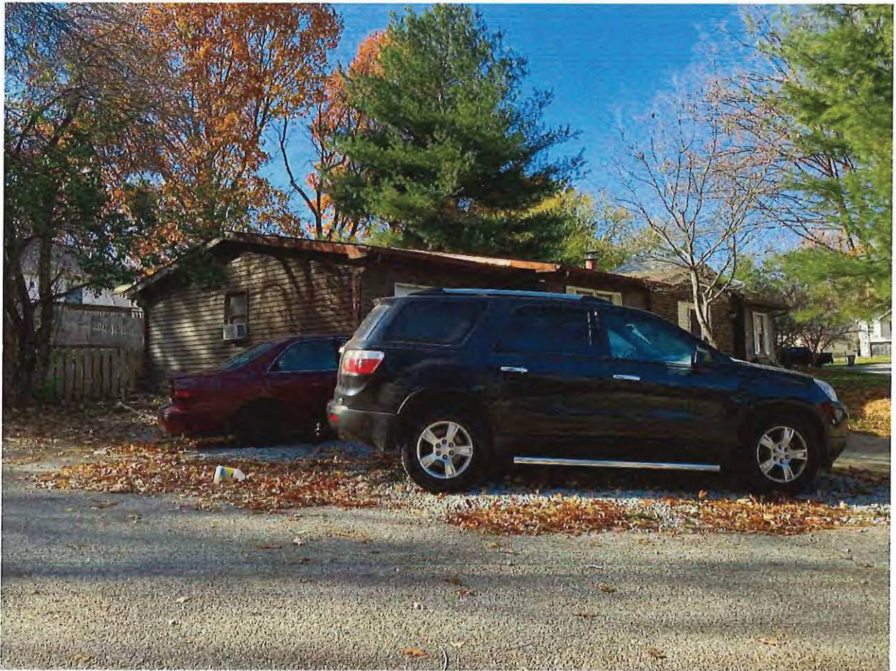
Photo 2: Driveway exceeding the allowed width on the northeast side of the property at 1205 W East Branch Drive on 11/09//2023.
