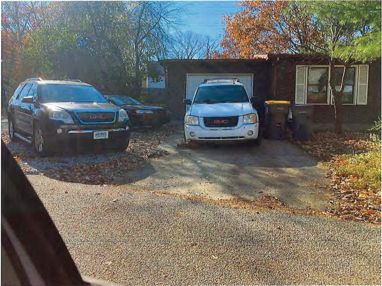
Photo 1: Driveway exceeding the allowed width on the northeast side of the property at 1205 W East Branch Drive on 11/09//2023.
