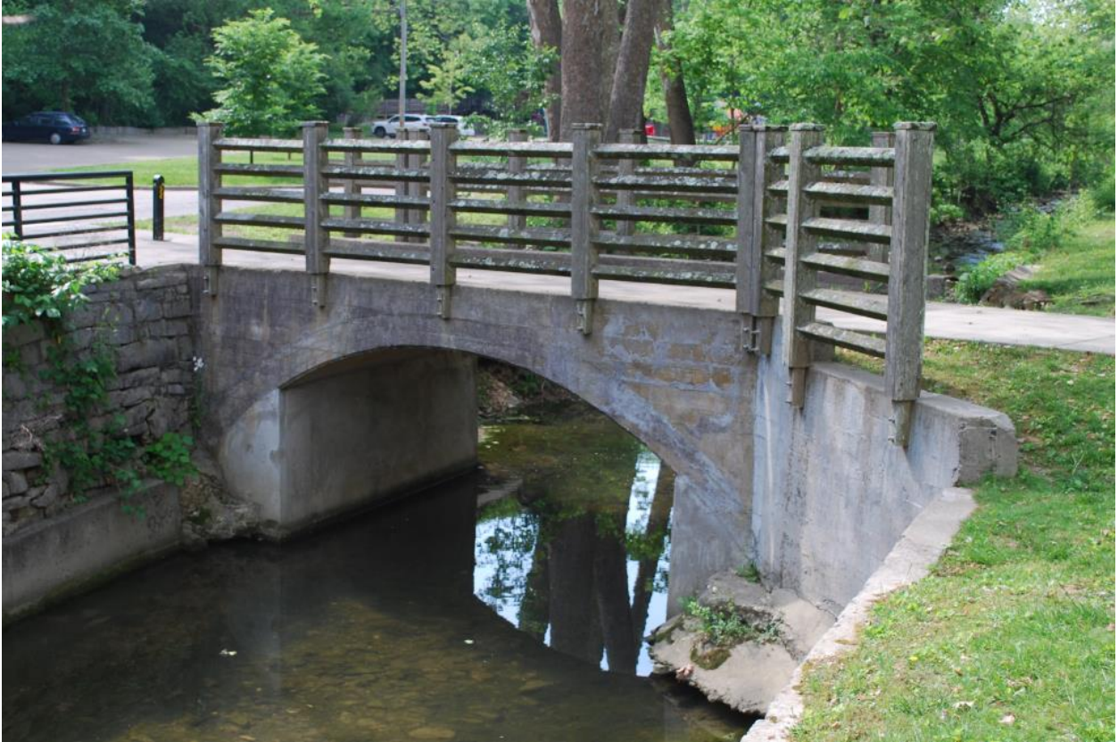
Image 8: Concrete Pedestrian Bridge, looking southwest
