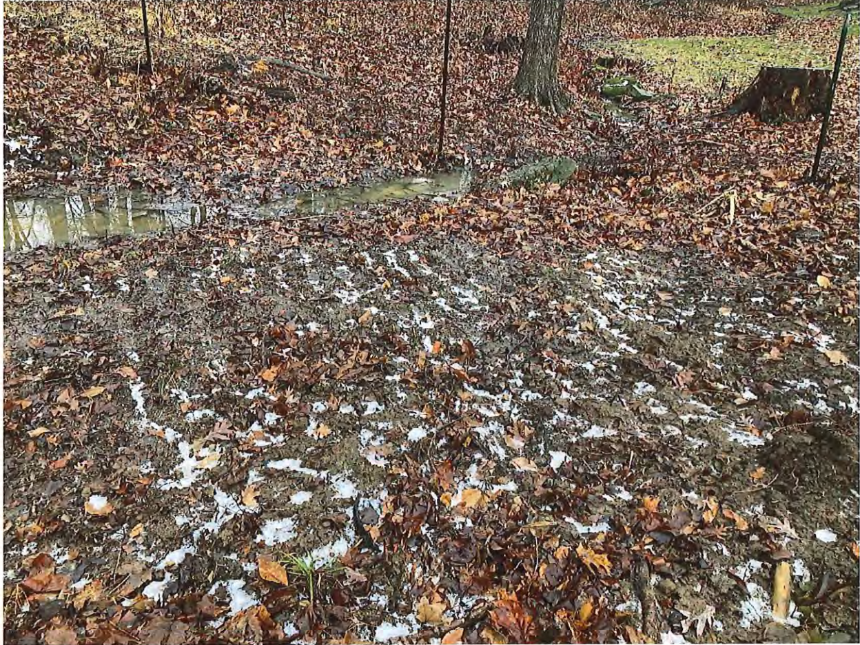
Photo 6: Intermittent stream, earth disturbance, absence of erosion control measures, and trees and vegetation removed near the intermittent stream (south-central area of the lot) at 2214 E Maxwell Lane on 01/23/2024, facing west.
