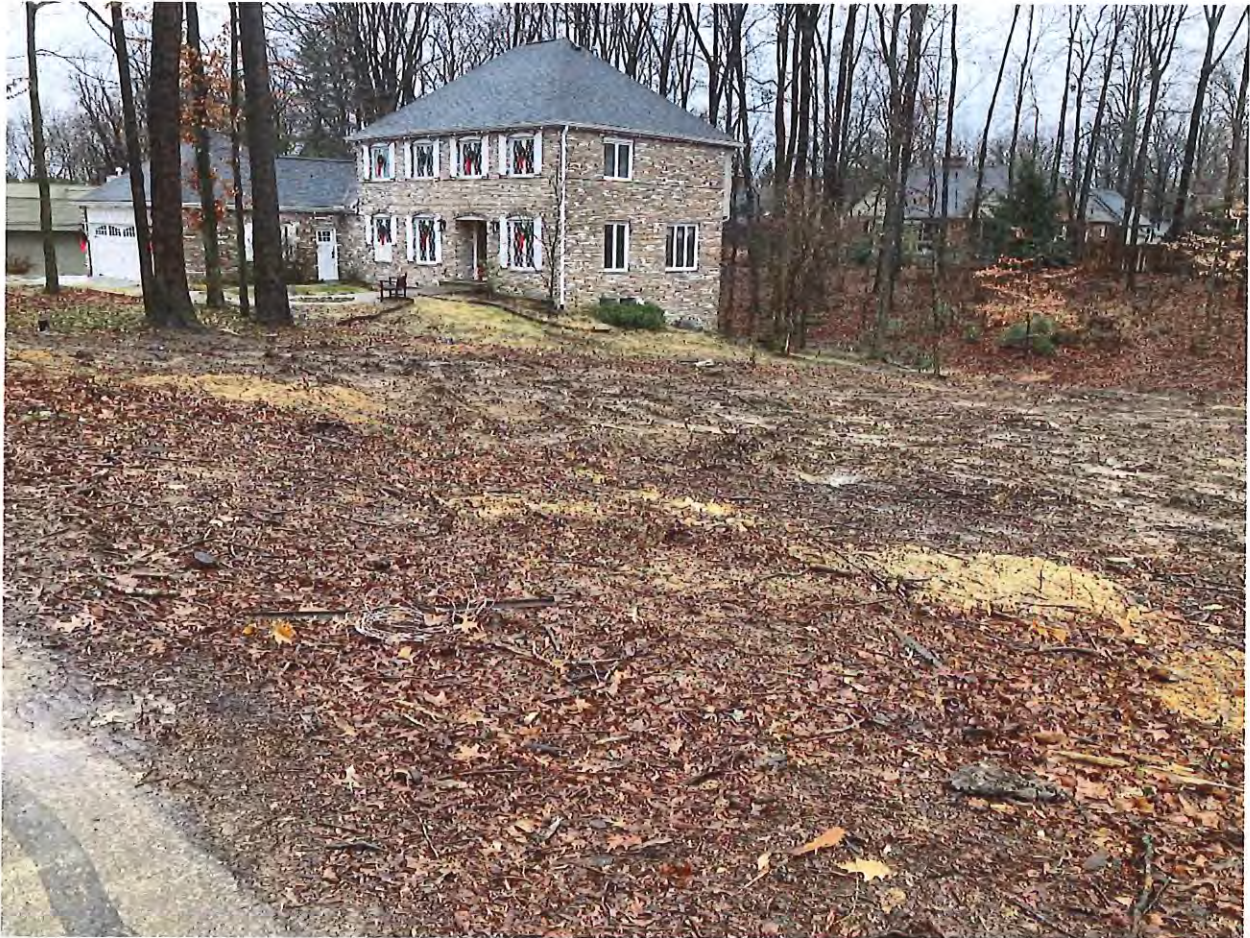
Photo 1: Earth disturbance, absence of erosion control measures, and trees removed on the northeastern side of 2214 E Maxwell Lane on 01/09/2024.
