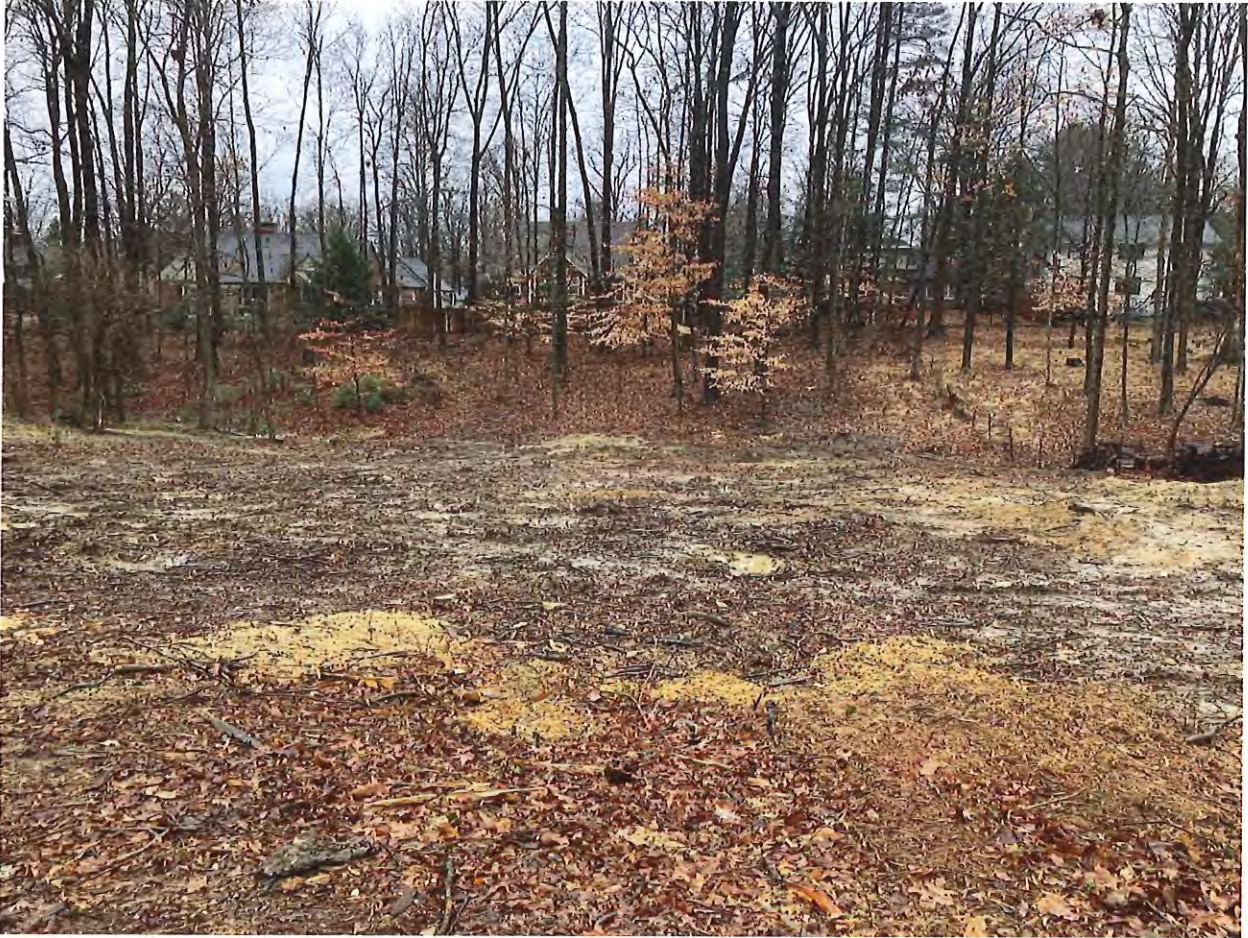
Photo 3: Earth disturbance, absence of erosion control measures, and trees removed at 2214 E Maxwell Lane on 01/09/2024 from the north, facing south.
