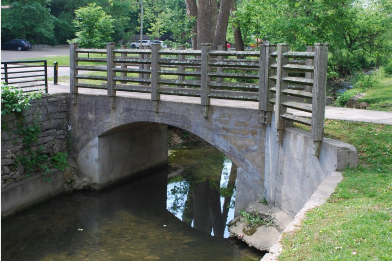
Image 8: Concrete Pedestrian Bridge, looking southwest
