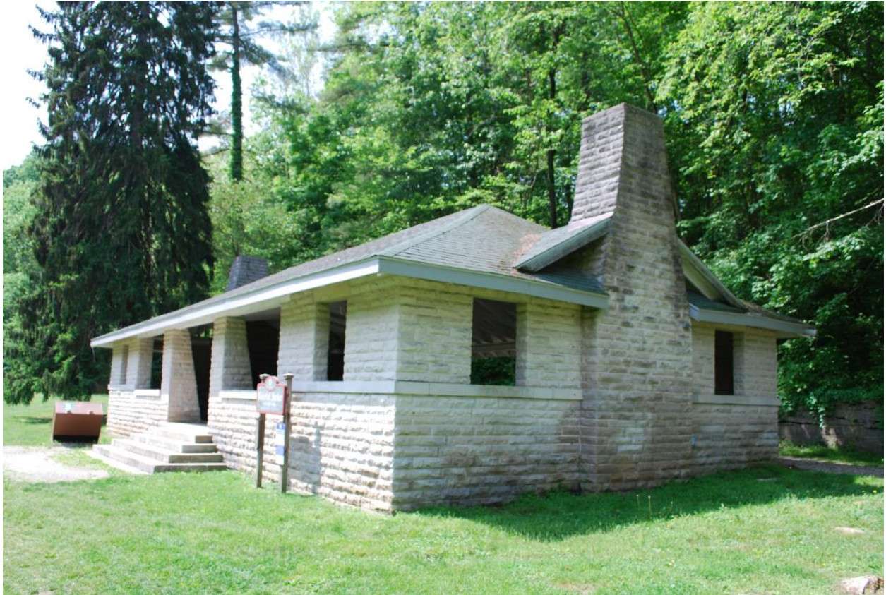
Image 4: Waterfall Cascades (Sycamore) Shelter House, looking southwest.
