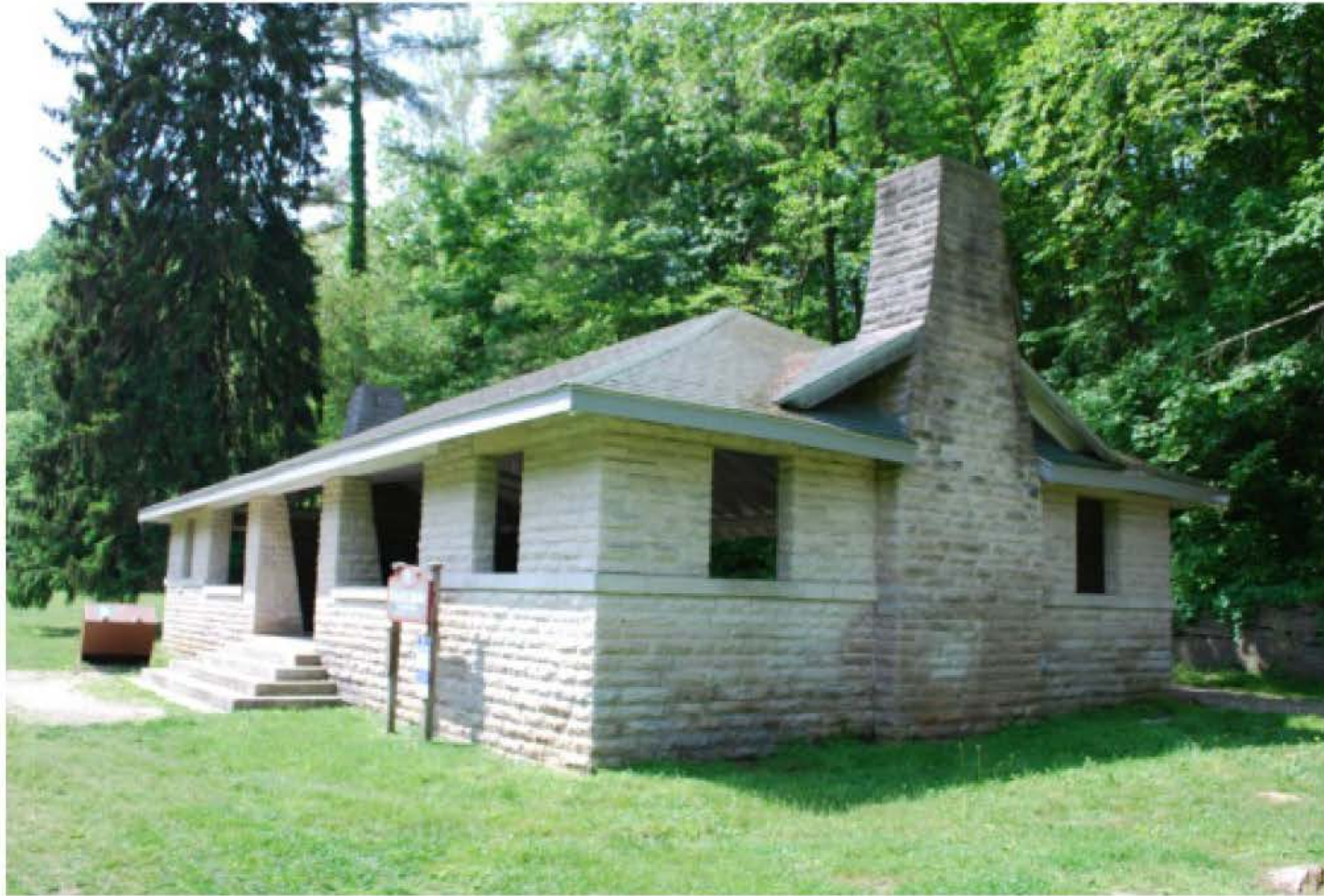
Image 3: Waterfall Cascades (Sycamore) Shelter House, looking southwest.
