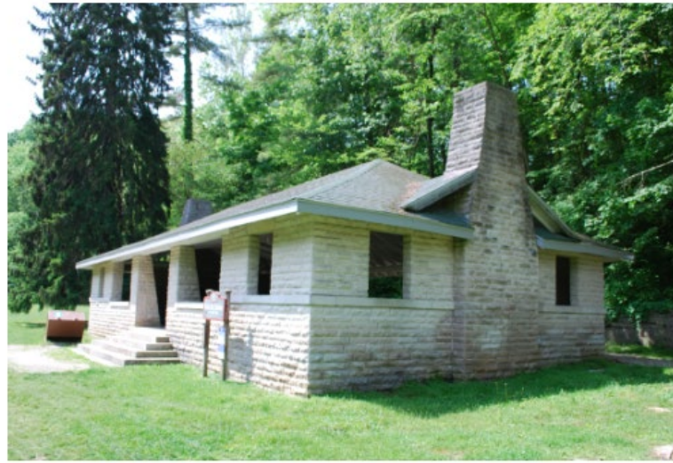
Image 3: Waterfall Shelter House, looking southwest.
