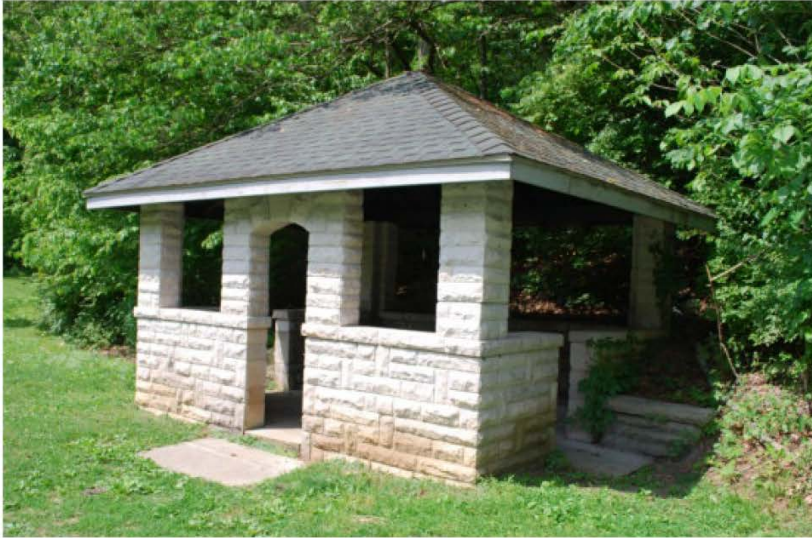
Image 5: Well House, looking southwest.
