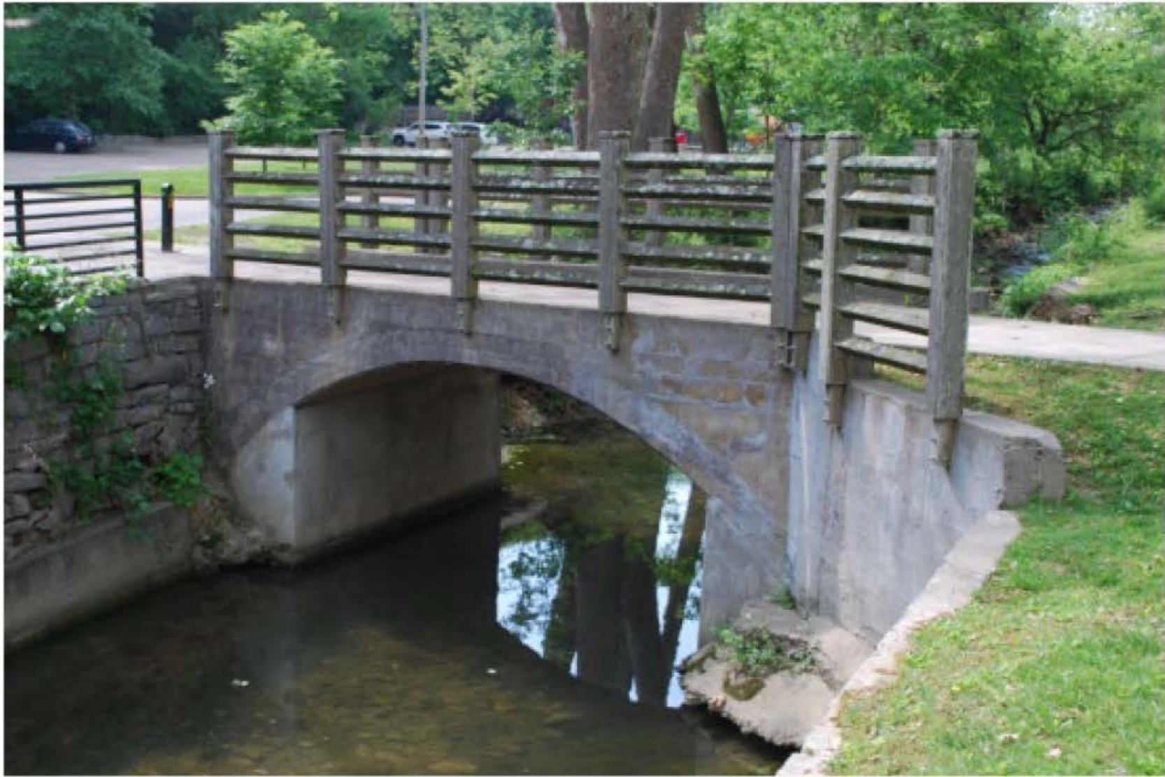
Image 7: Concrete Pedestrian Bridge, looking southwest
