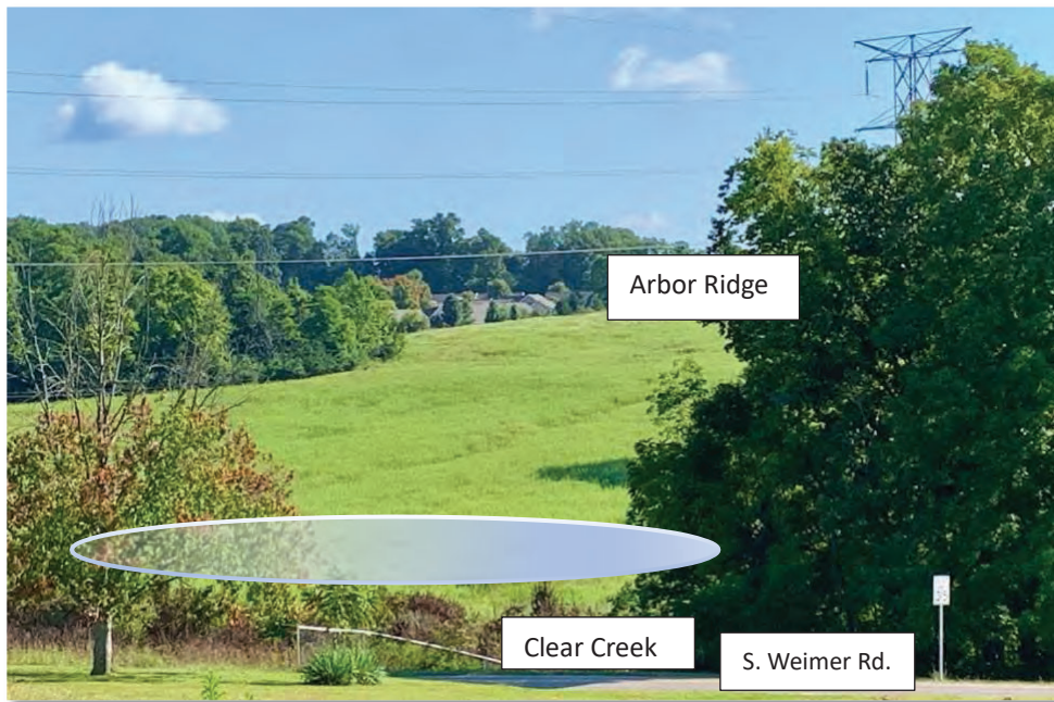
Figure 1. View of “Shasta Meadow” Hillside from 1812 Weimer Road. Photo by T. Frick, 9/03/2023. Possible location of proposed Weimer Retention Pond and text annotations are superimposed (also see Figure 2). Clear Creek is not visible here because of the steep slopes along the riparian buffer.
