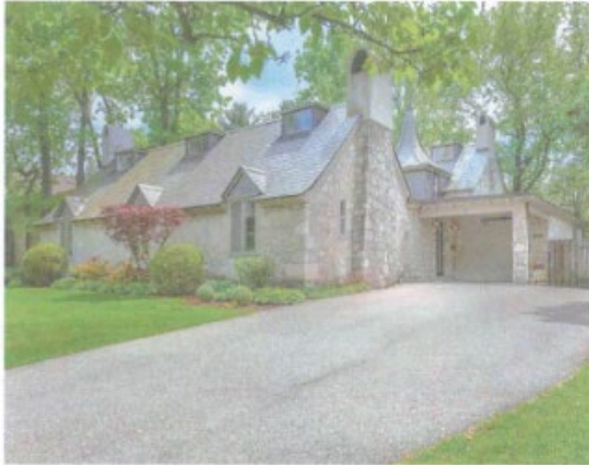
Exterior of home before renovation.
