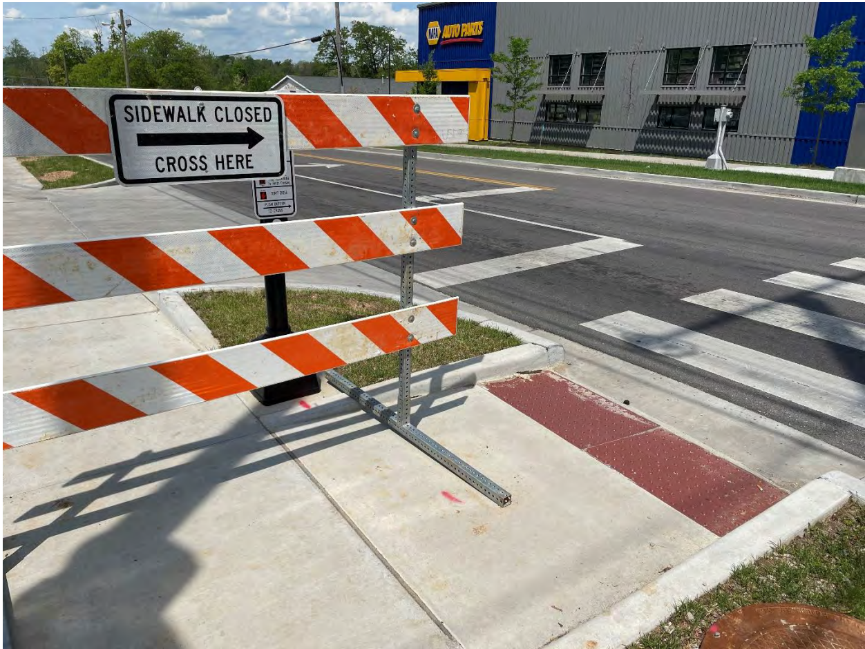
Photo 2: Sidewalk curb ramp and pedestrian push button blocked by sidewalk closure signage at W 17 th St and N Madison St (5/2/2024)
