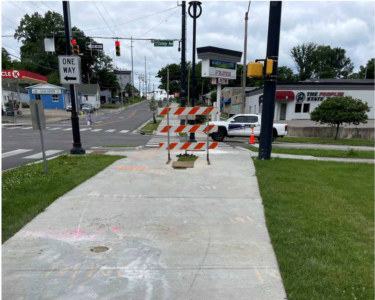
Photo 11: Sidewalk closure that is not sufficient to close the sidewalk for the work in the area. The barricade does not properly close the sidewalk sections and can be missed by visually impaired pedestrians. (5/29/2024)
