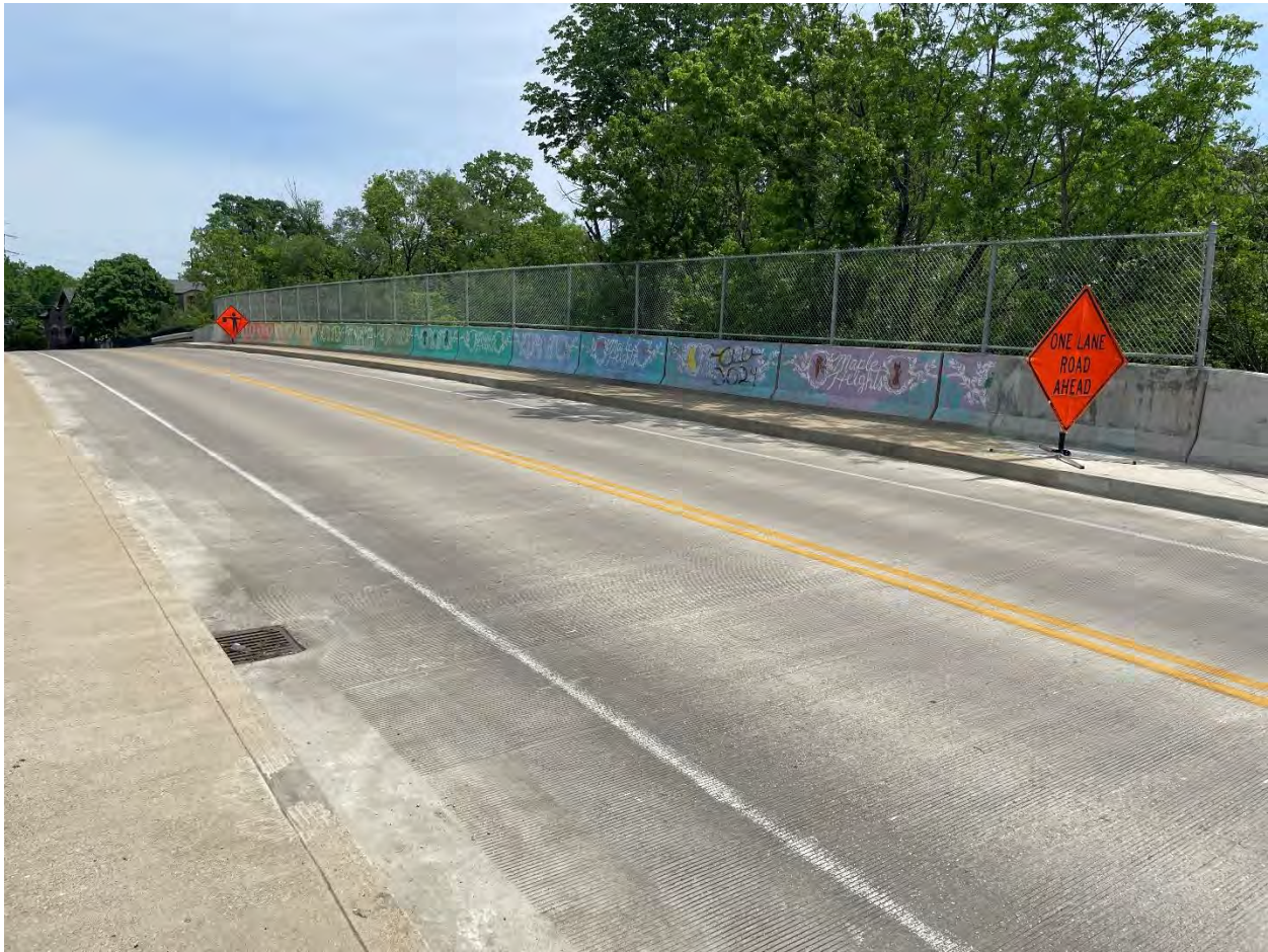
Photo 7: Signage blocking the sidewalk along N Madison St between W 14 th St and W 11 th St on the bridge. Signage is to be placed in such a way to maintain a 4 ft clear path for sidewalk usage. (5/8/2024)
