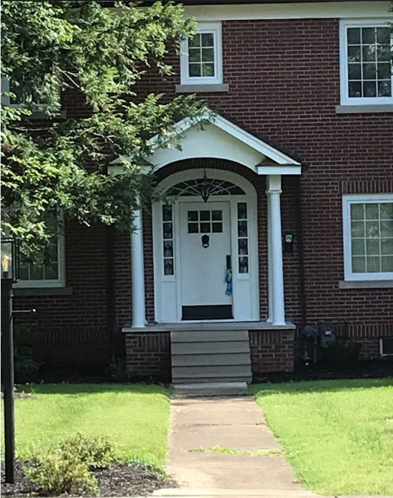
Current entrance with replacement door and limestone steps
