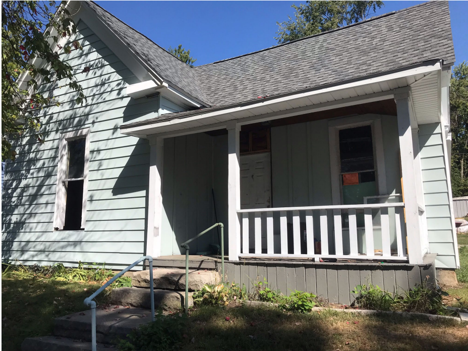
Porch after alterations
