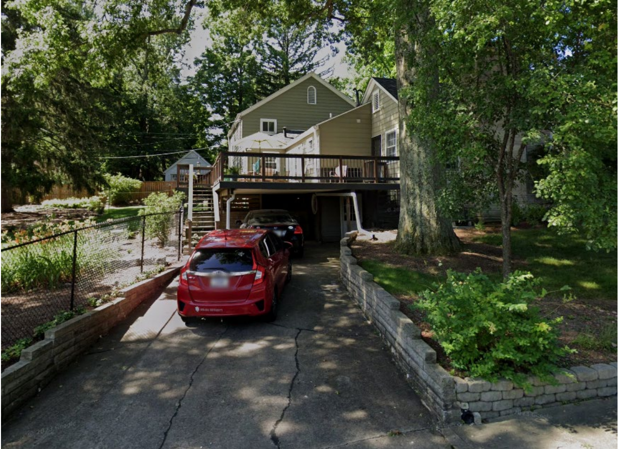
Deck prior to damage
