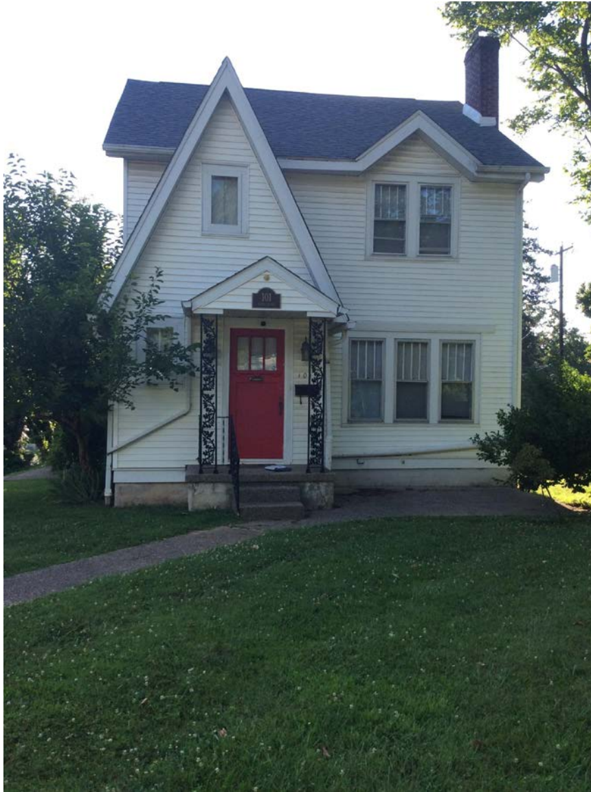
101 N Bryan Avenue – Contributing Architectural Style: English Cottage, 1925
