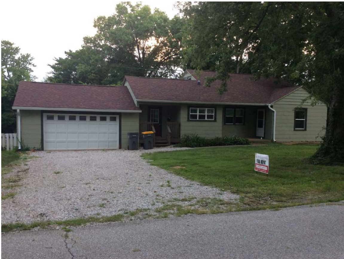
121 N Bryan Avenue – Contributing Architectural Style: American Small House, 1949 (Severely altered)
