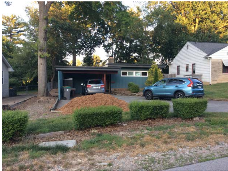
201 S. Hillsdale Drive, the first home Elaine Doenges designed
