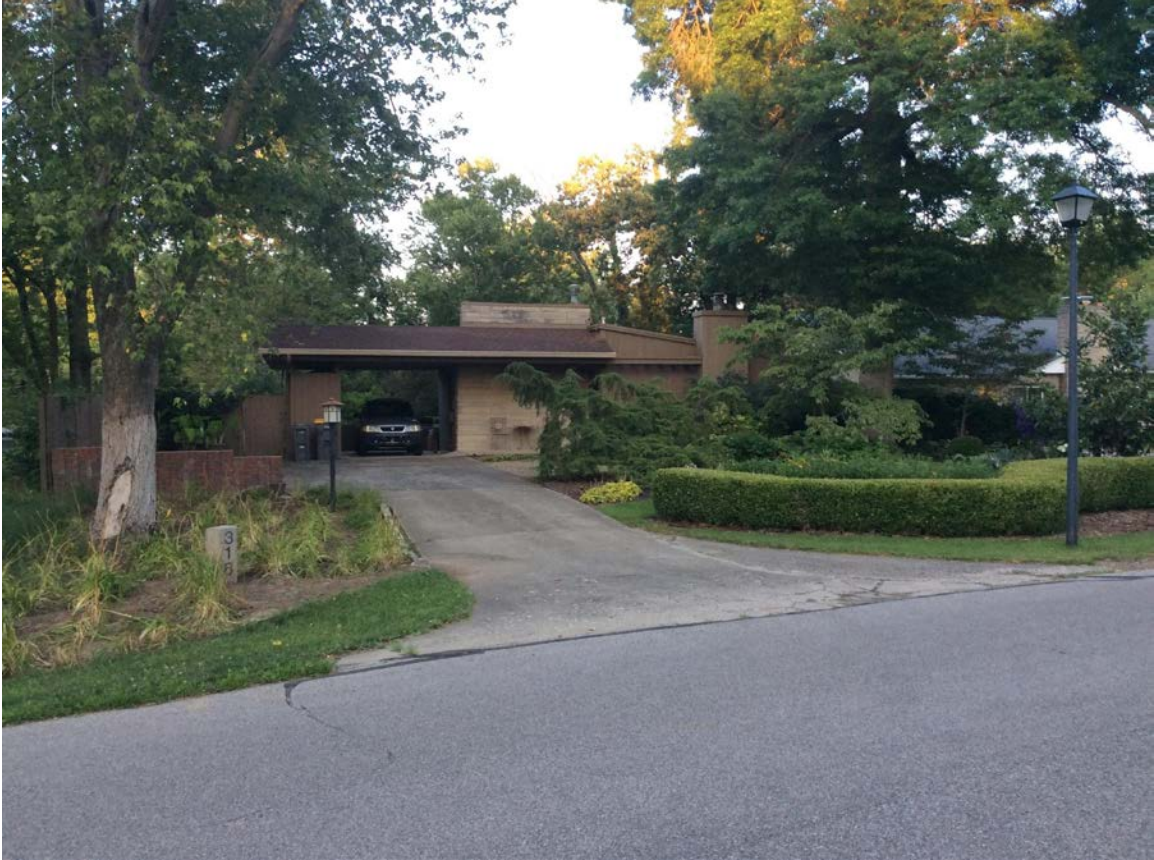
316 N Hillsdale Drive – Notable Architectural Style: Massed Ranch, 1955
