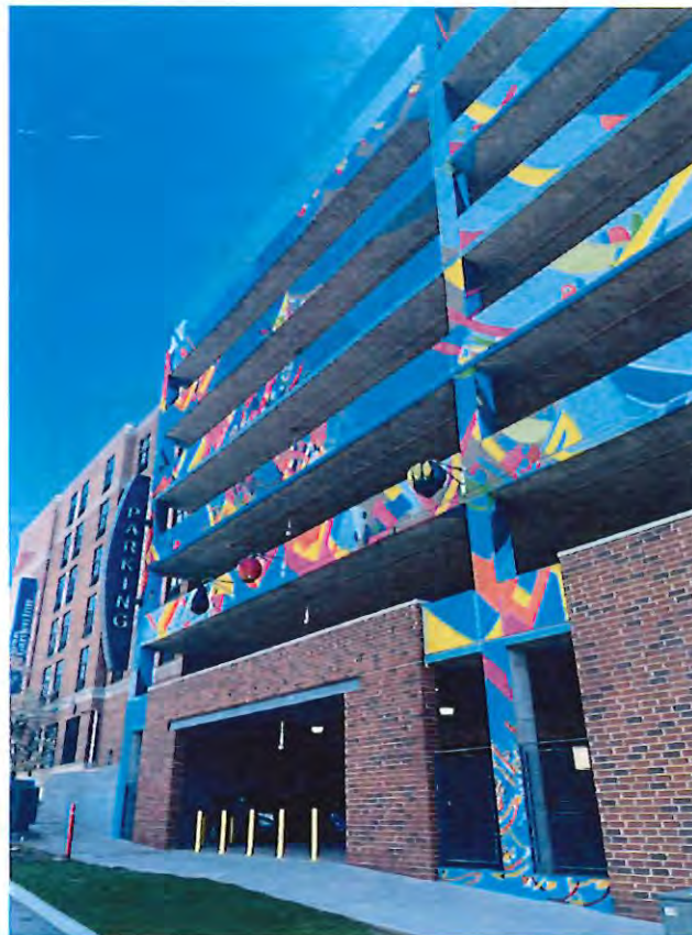
Figure 3: Morton Street Parking Garage – view from 7 th Street
