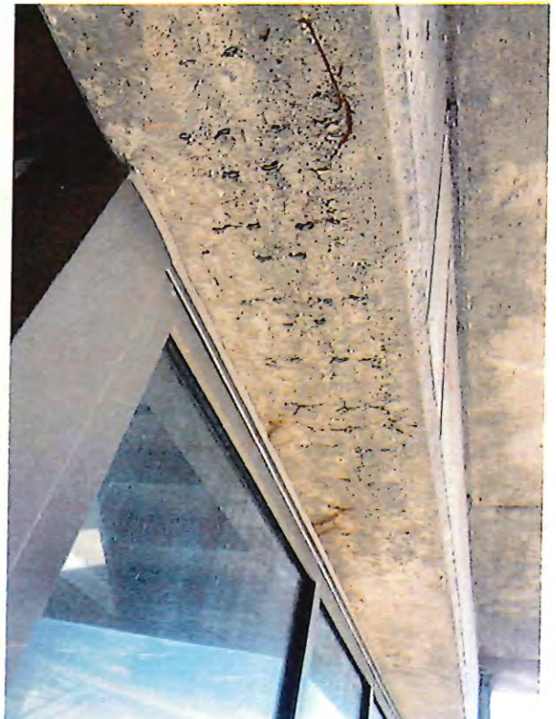
4 - beam cracks.JPG
