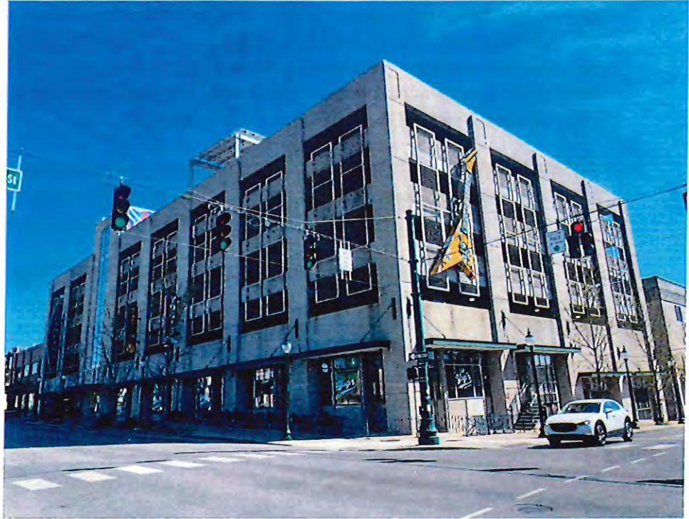
Figure 1: Walnut Street Parking Garage – view from Walnut/7 th Street intersection
