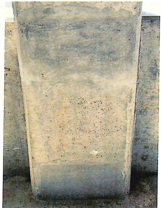
12 - delaminated column repair.JPG
