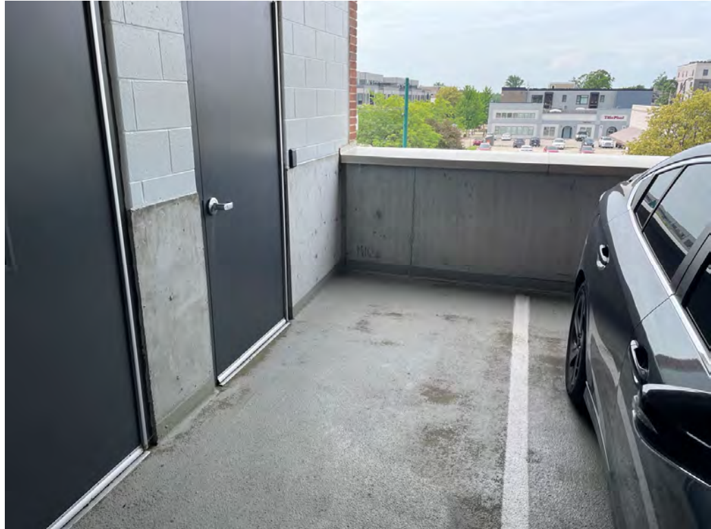
Photo 03: Exterior view of IT room door
