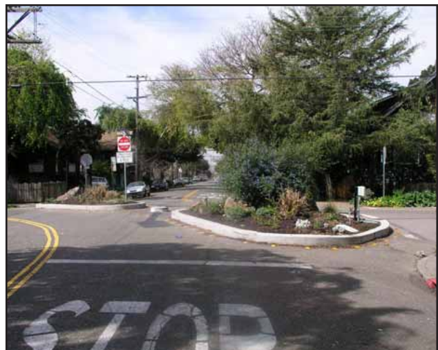
Bicycle Boulevard traffic diverters in Berkeley, CA
