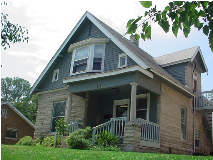
View from College Street façade looking southwest, showing modern porch balustrade.
