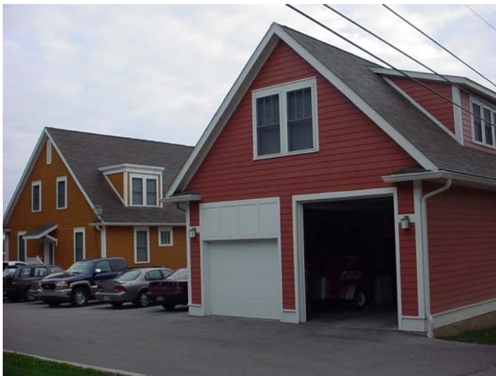
View from alley looking northeast, showing new construction. Only the structure in the foreground is a part of the designation.
