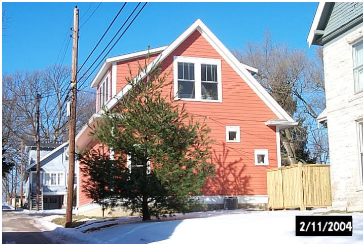
The newly constructed carriage house (depicted) is located on the south west corner of the lot.
