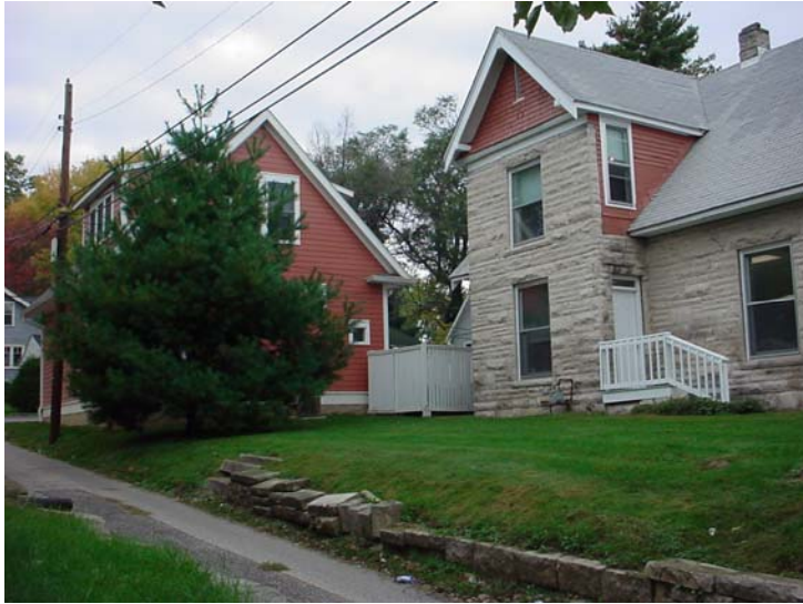
Area where porch restoration could occur, showing compatible new construction
