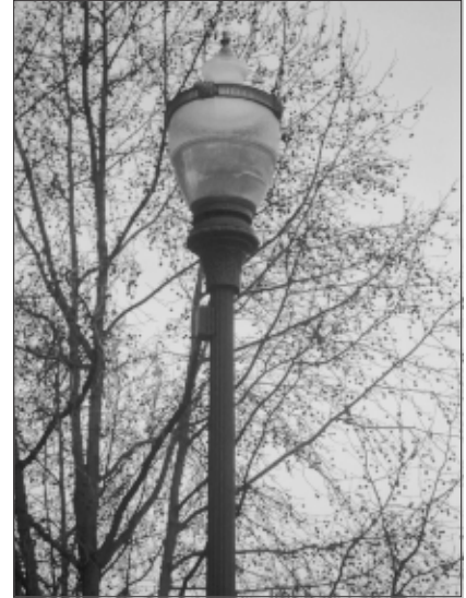
The light fixtures and poles should be unifying design elements that promote visual interest and variety.
