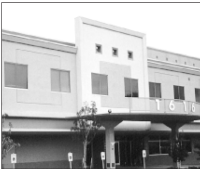
Stucco that is detailed to convey a sense of scale and provide visual interest is an appropriate material treatment. (Boulder, CO)
