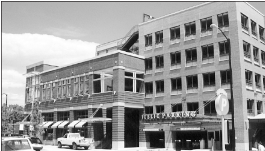
A part of this infill building is a parking structure that is set back from the front and sides of a retail wrap. The openings in the parking section reflect window proportions similar to those seen historically in the area. (Boulder, CO)
