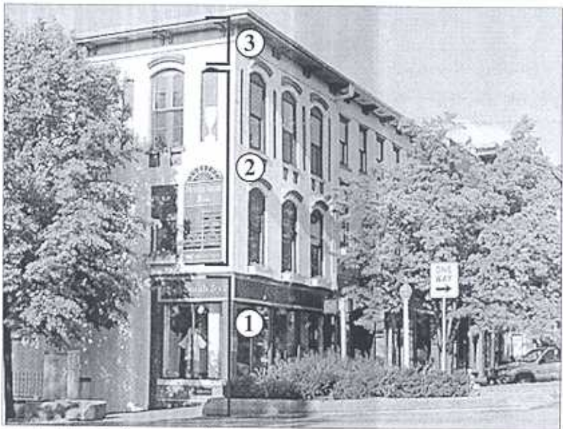
This building in Downtown Bloomington incorporates the basic building blocks: (1) base, (2) middle and (3) cap. (Bloomington, IN)
