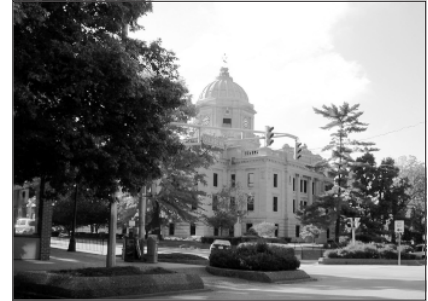
The Courthouse Square serves as the center of the Courthouse Square. (Bloomington, IN)
