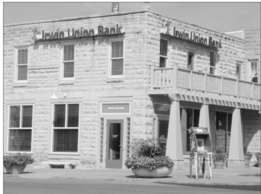
Limestone has been used historically throughout the commercial core of Bloomington. Masonry, including both stone and brick, is preferred for new construction. (Bloomington, IN)
