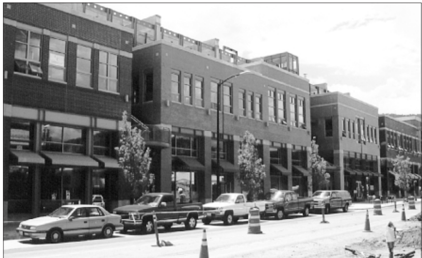
This single infill building is divided into smaller building modules that reflect traditional building widths. Upper floors step back from the front, thus maintaining the traditional two-story scale of the street. (Boulder, CO)
