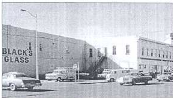
The street wall is broken with a vacant lot. (Boulder, CO)
