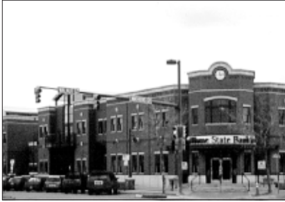
Divide a larger building into modules, such as this, to reflect traditional building widths.
