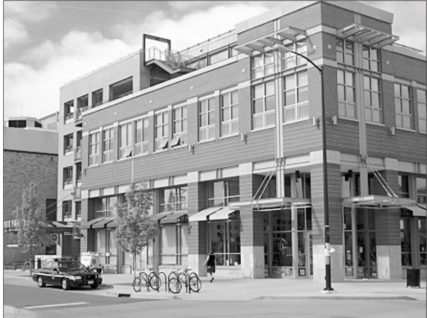
A part of this contemporary infill building is a parking structure which is concealed with a “wrap” of office and retail uses. The openings in the parking section of the development also utilize window proportions similar to those seen historically. (Boulder, CO)
