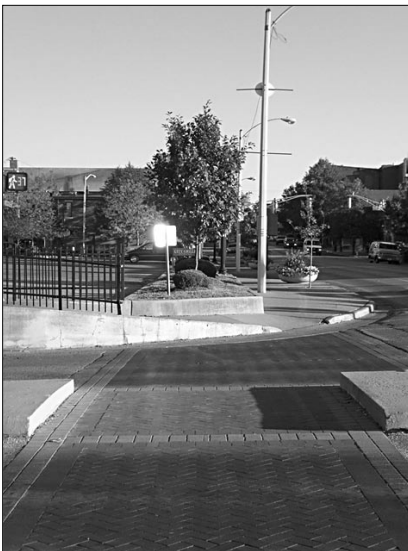
3rd Street and South College Avenue intersection. Embellished crosswalk leads to poorly configured handicap ramp. (Bloomington, IN)
