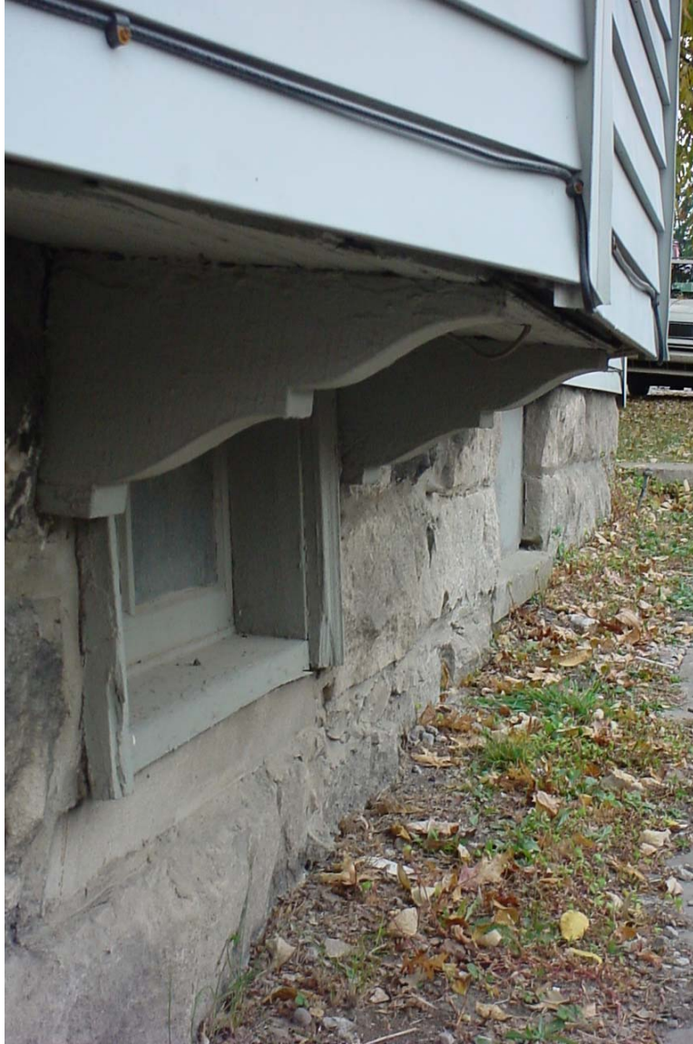
Curvilinear Brackets beneath Eighth Street Bay
