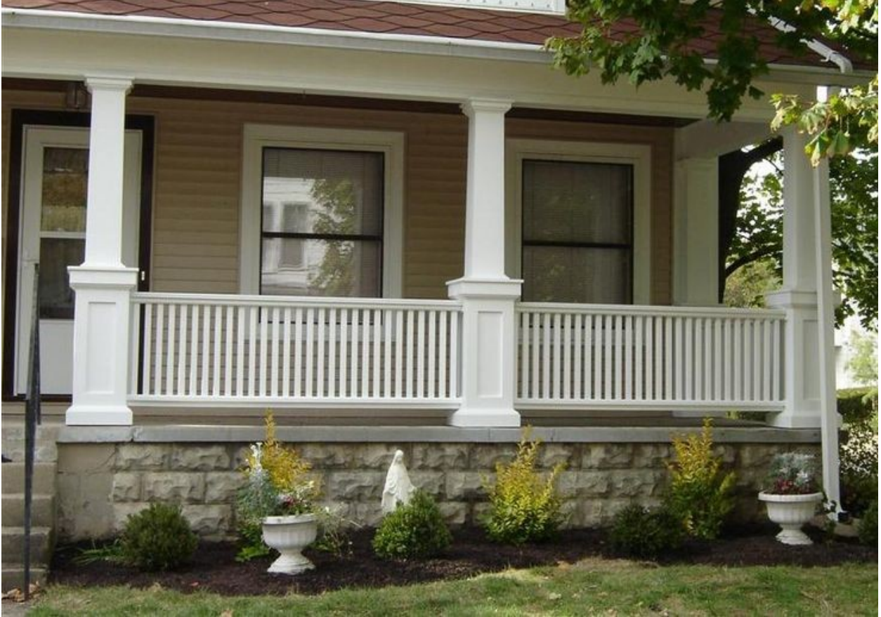
Example of replacement porch post style recommended by BHPC staff.
