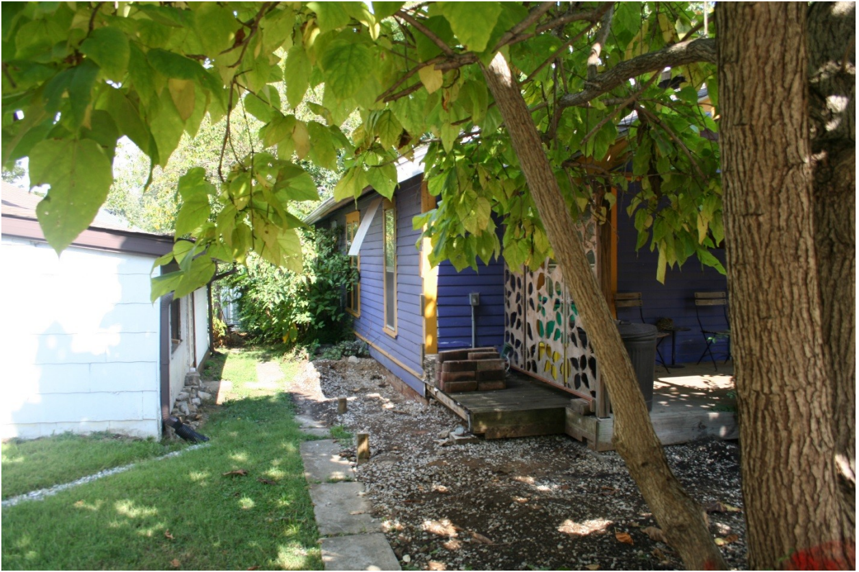
South and west sides, looking NE
