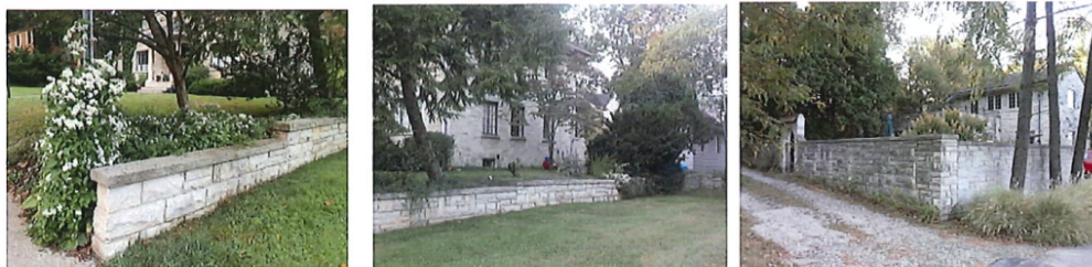
Retaining wall on north side
