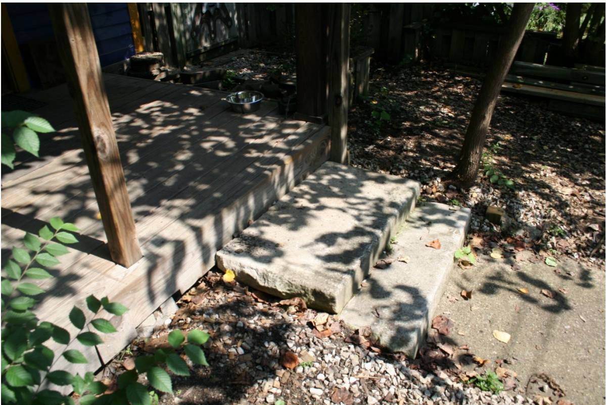
Front stoop and existing front porch deck, to be demolished
