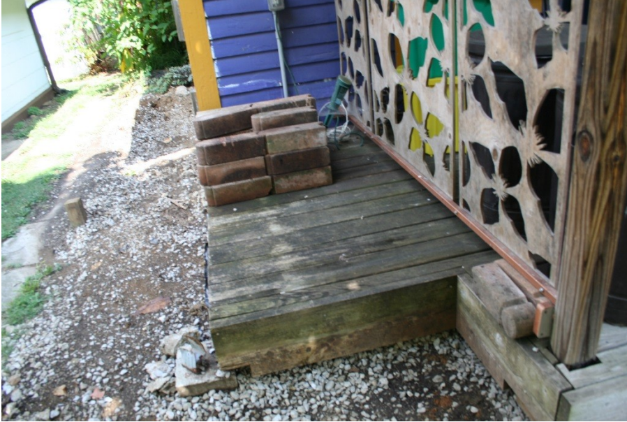
Protruding west section of front porch, to be demolished
