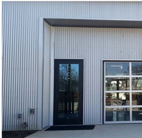
CORRUGATED METAL PANEL - VERTICAL
