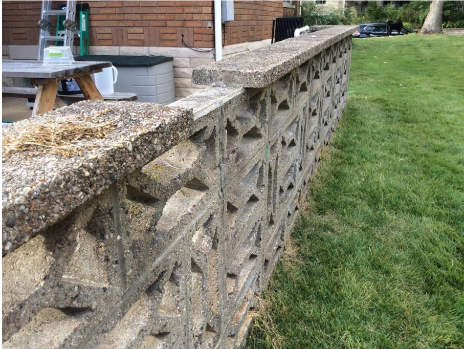
Figure 2: East side of block wall, looking NW
