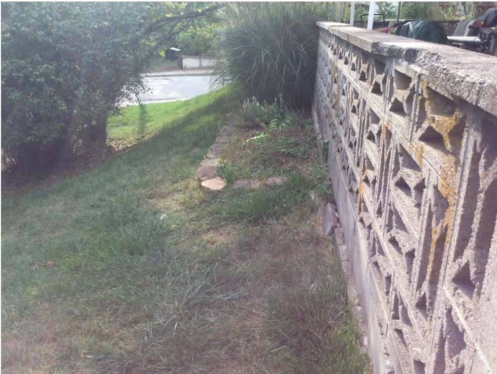
Figure 3: South side of wall, looking east
