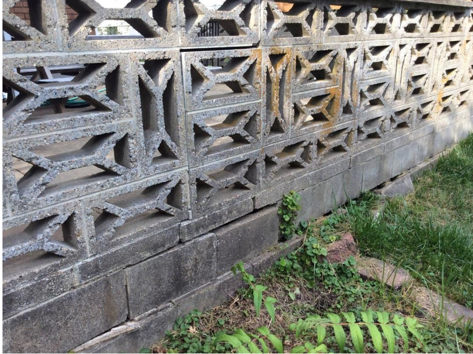
Figure 4: Close-up, south side of wall, looking NE
