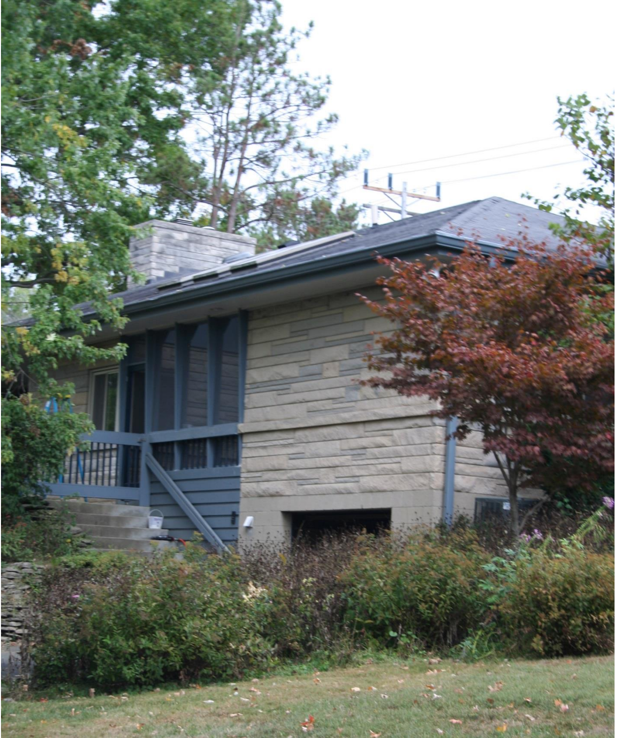
Figure 1: Progress as of October 4, 2017
