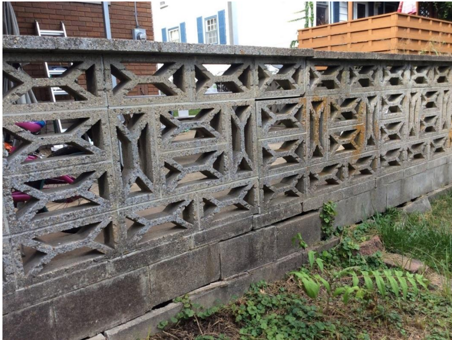
Figure 5: South side of wall, looking NE
