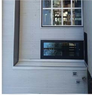
CORRUGATED METAL PANEL - VERTICAL
