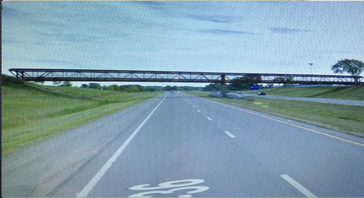
MARYSVILLE, OHIO US-33 COST (2015): $1.6 MILLION
