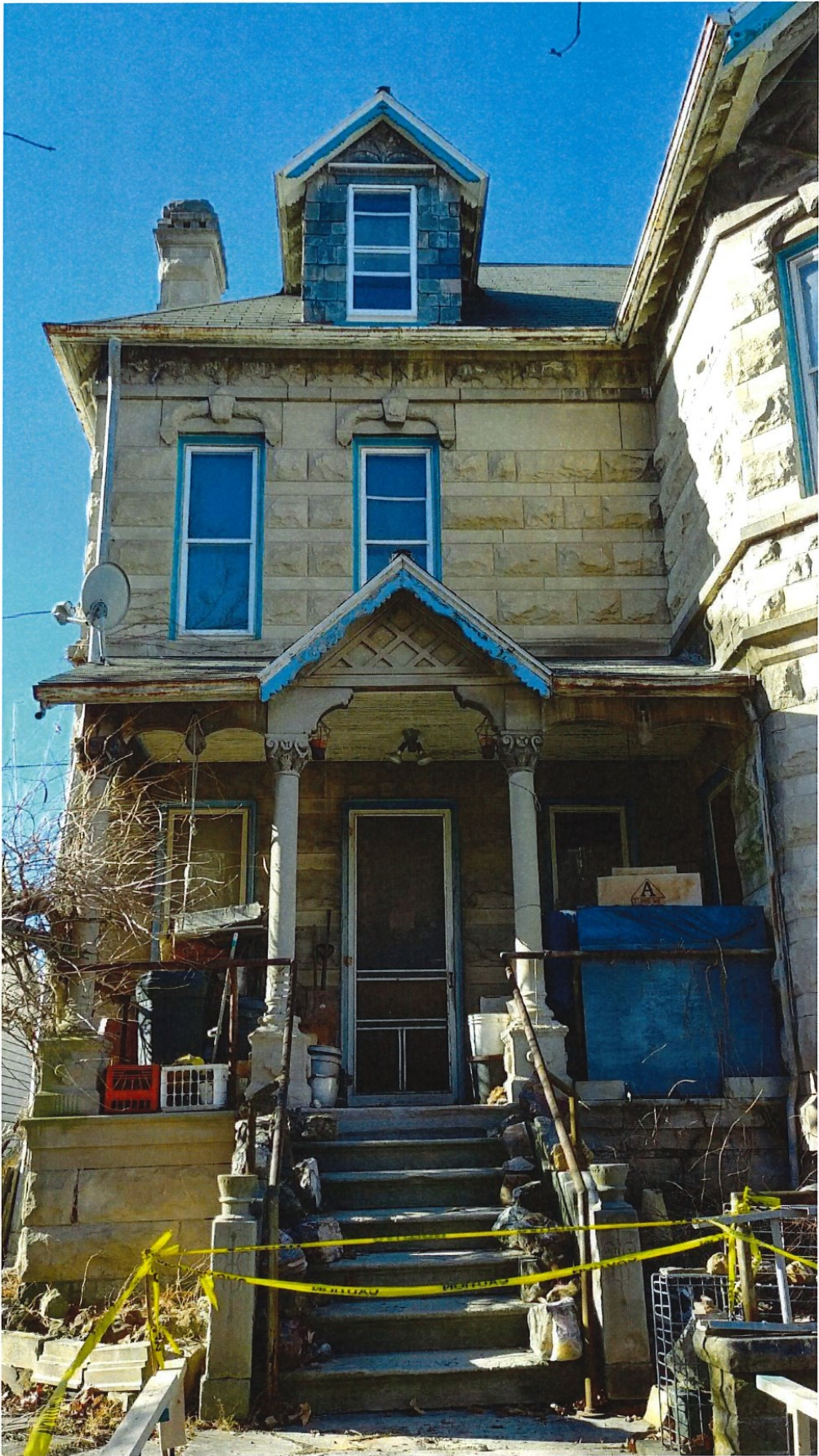
East elevation rear porch and second story
