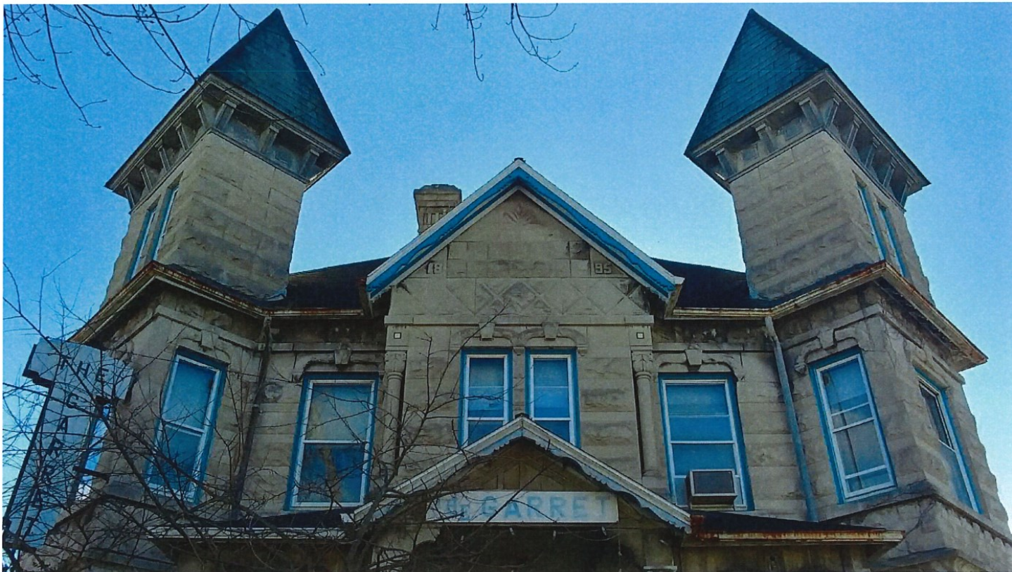
North facade limestone detailing
