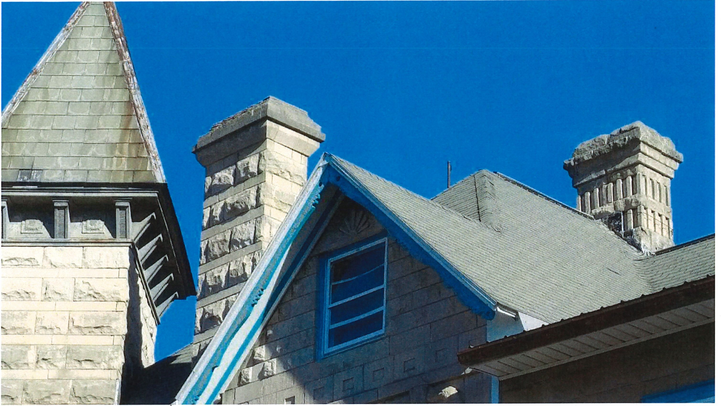
Limestone chimney detailing and West gable detailing
