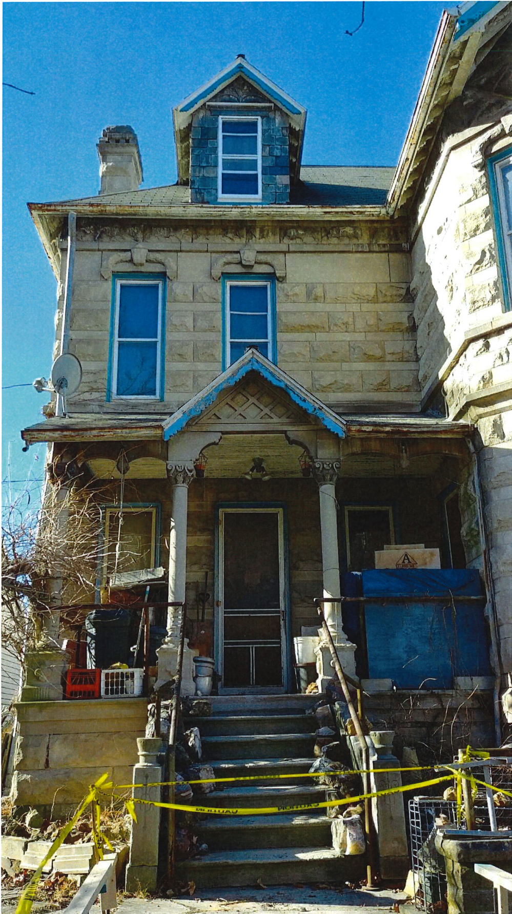
East elevation rear porch and second story
