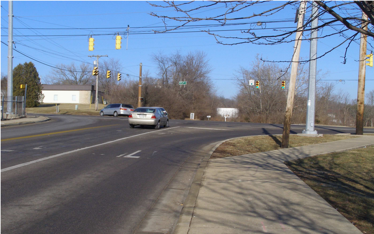
Patterson Drive looking northbound towards W. 3rd Street (~40 feet).
