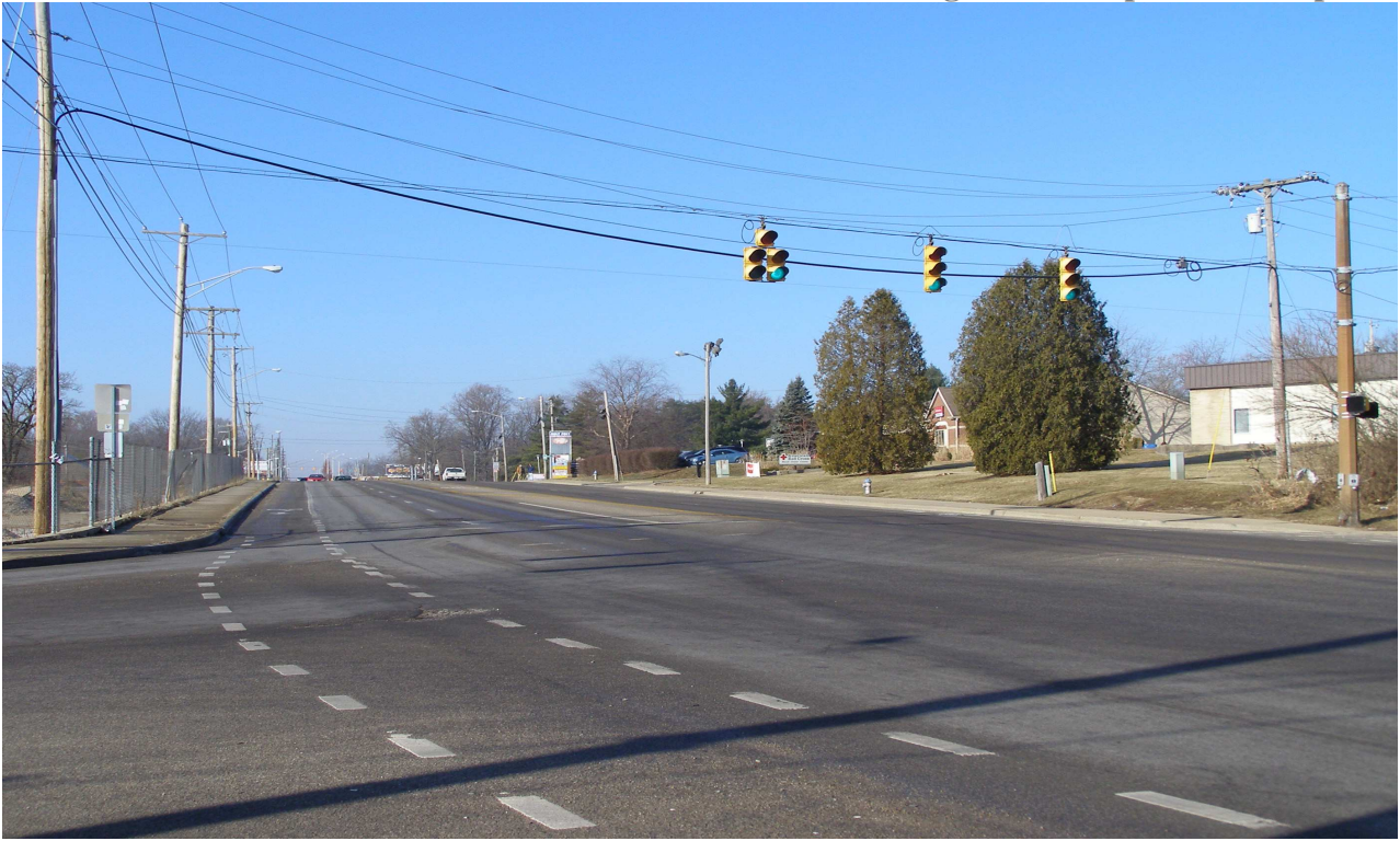
W. 3rd Street looking west from the intersection of Patterson Drive (~60 feet).
