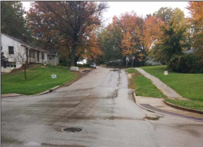
Hillsdale Drive looking south towards 3 rd Street
