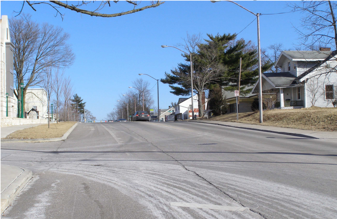
E. 3rd Street looking eastbound at S. Rose Avenue (~30 feet).
