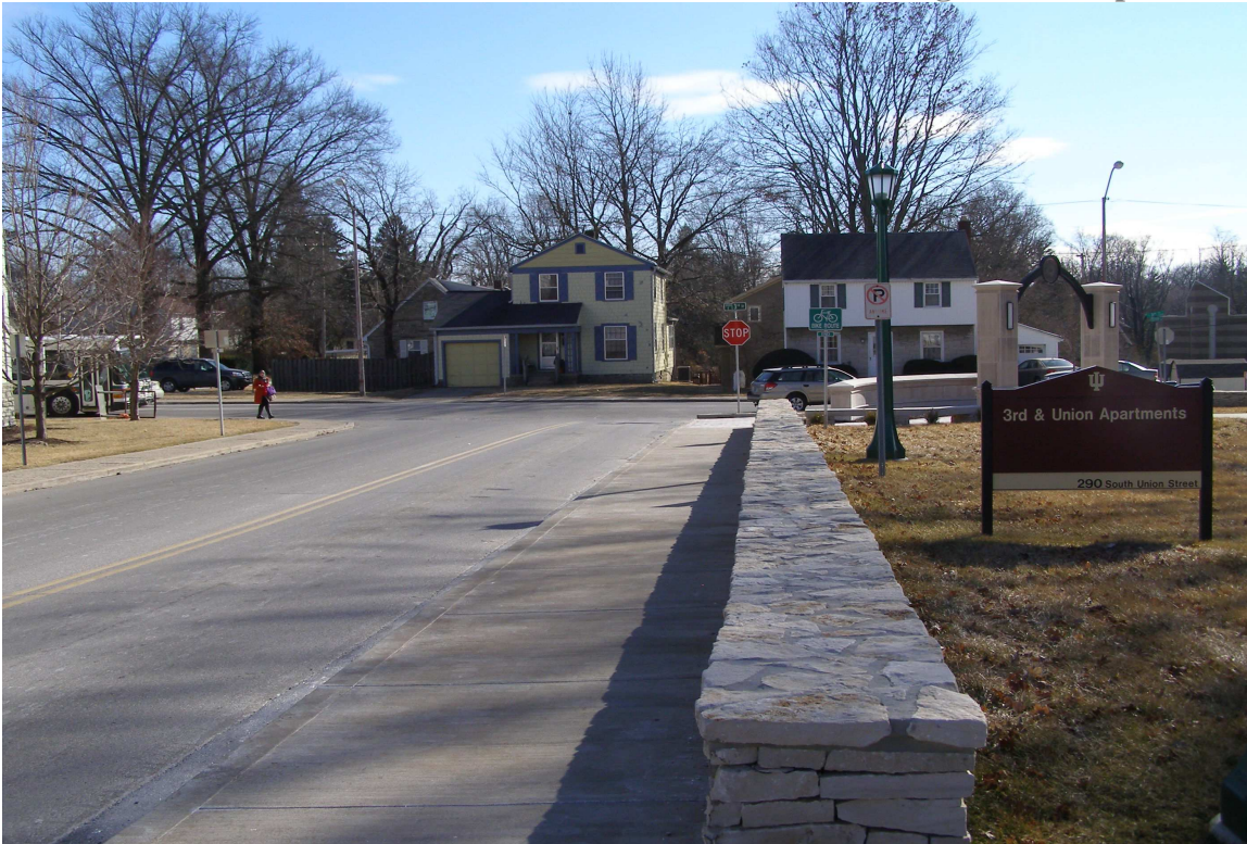
S. Union Street looking southbound towards E. 3rd Street (~30 feet).
