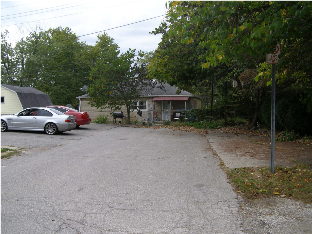
The dead-end of E. 4 th Street (~20'), with the paved pull-off parking areas of 2408 (left) and 2401 (right).
