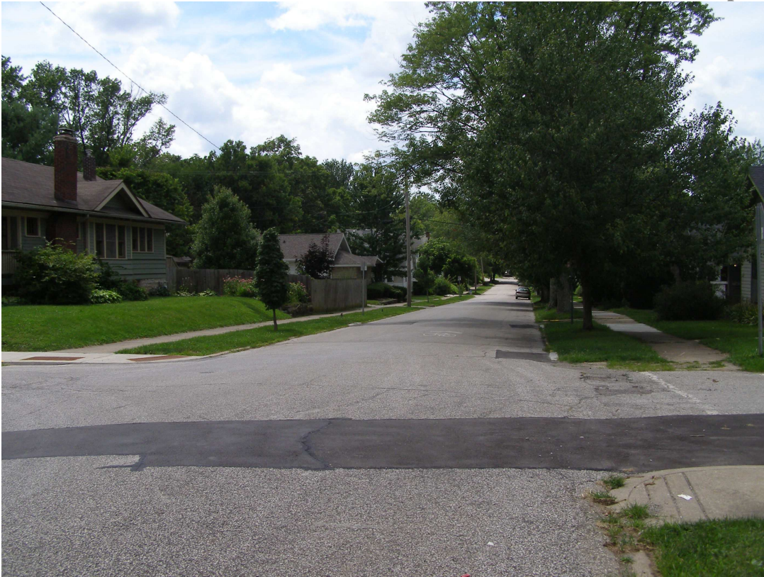
Looking west on E. 12 th Street (~24') at the intersection with N. Lincoln Street.
