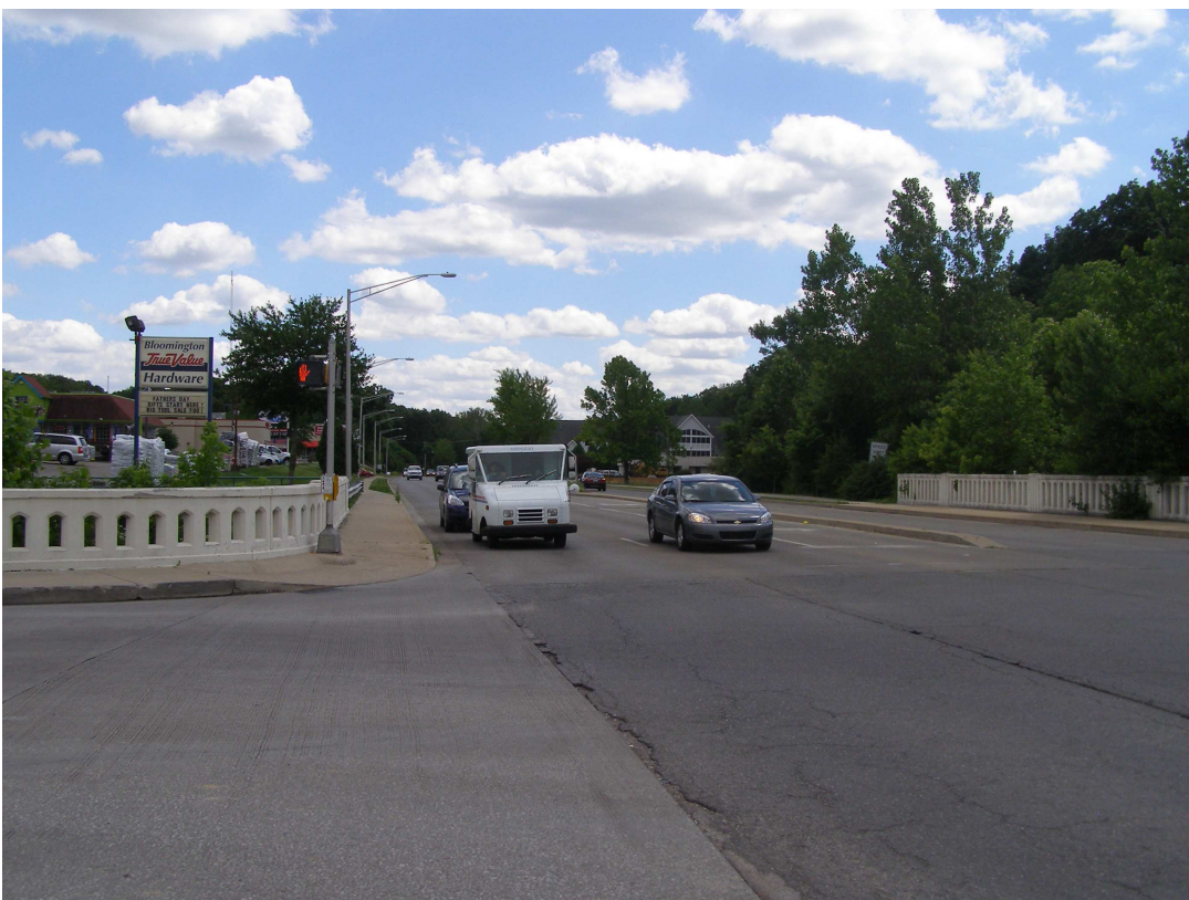
Looking south on S. College Mall Road (~70') from the intersection with E. Covenanter Avenue.
