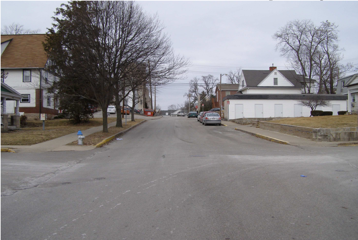
Fess Avenue looking northbound at the intersection with E. Hunter Avenue (~25 feet).
