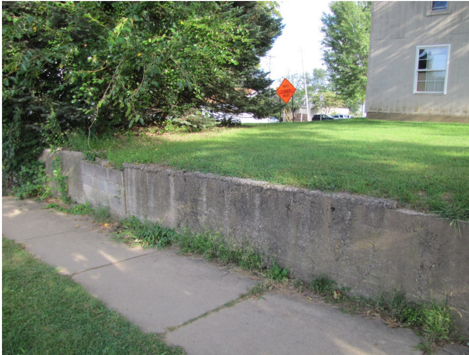
Close up of existing concrete/block wall to be mostly removed.
