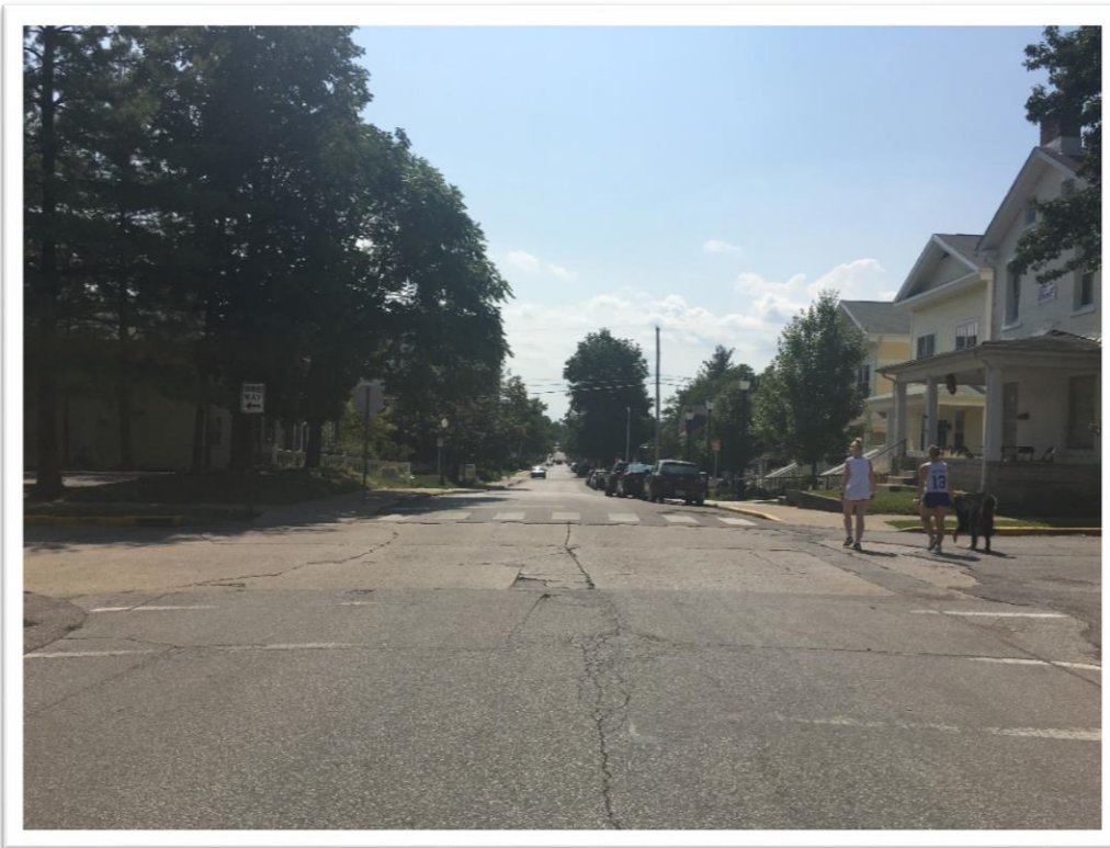
Looking south on Grant towards the intersection with 8th Street.
