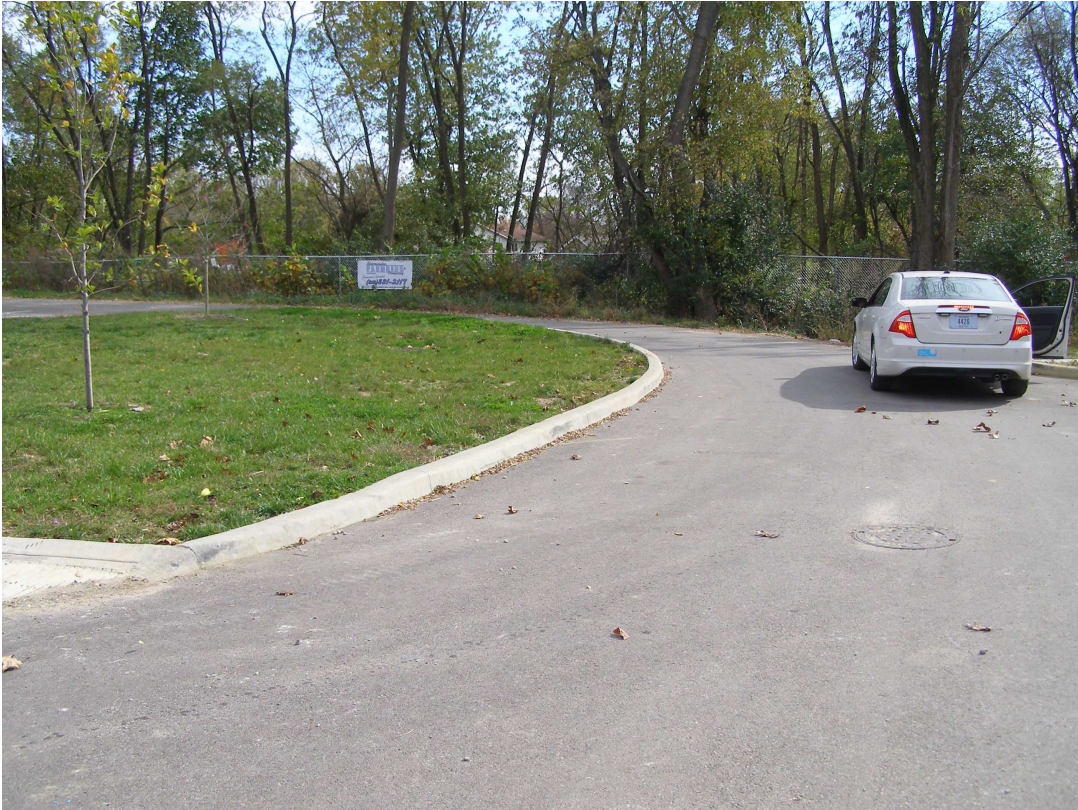
The second curve on the west side of W. Moravec Way (~19). The proposed no parking zone is on the left side of the photo.
