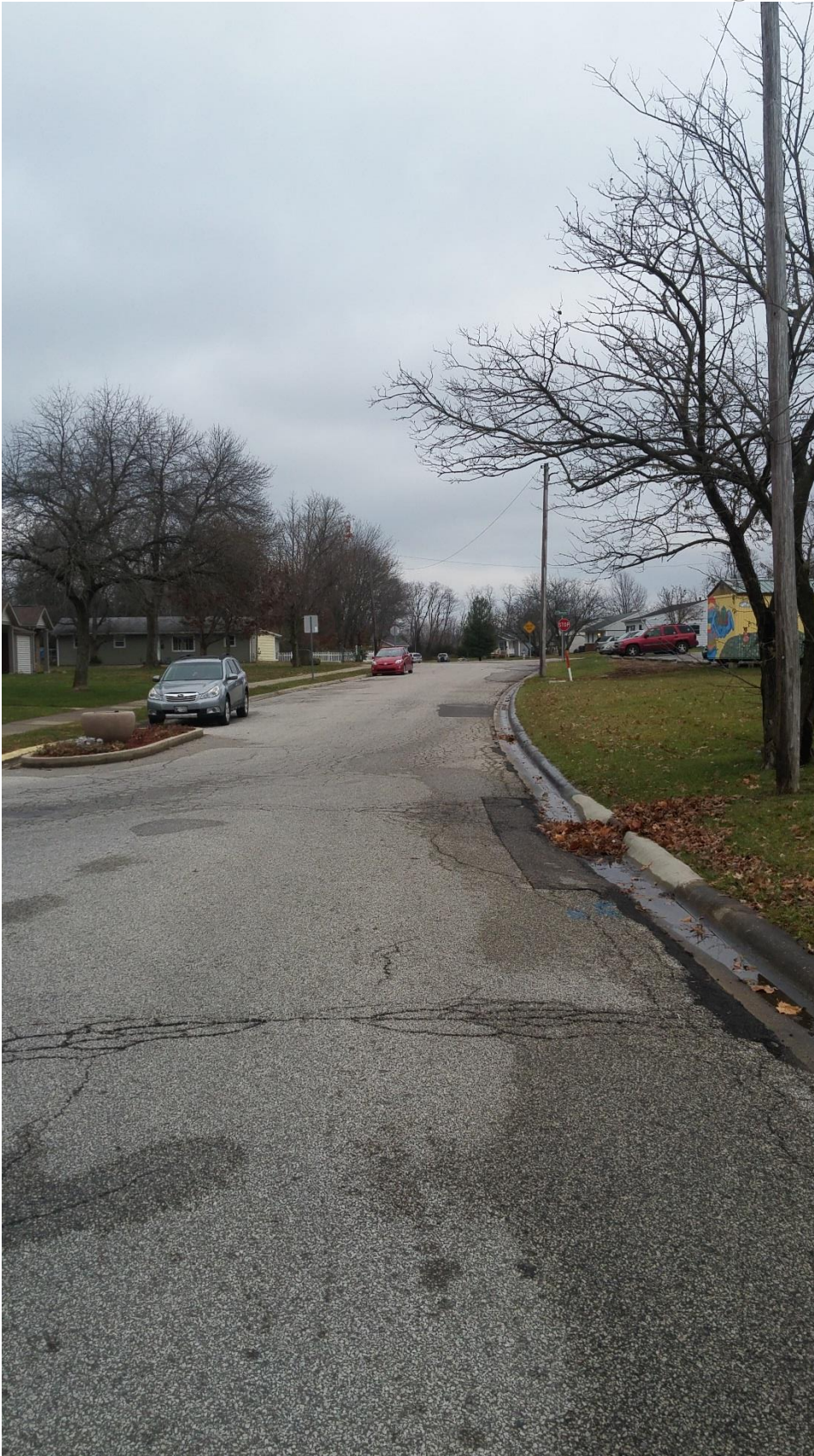
Existing conditions looking east along 12 th Street toward Monroe Street
