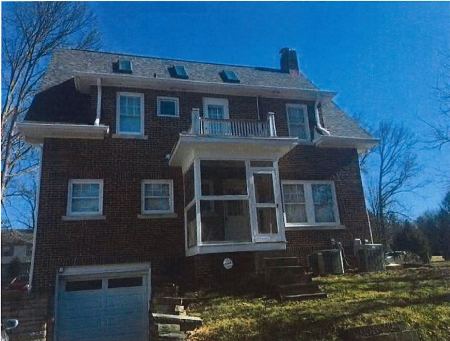
West elevation – screened porch and garage door to be replaced
