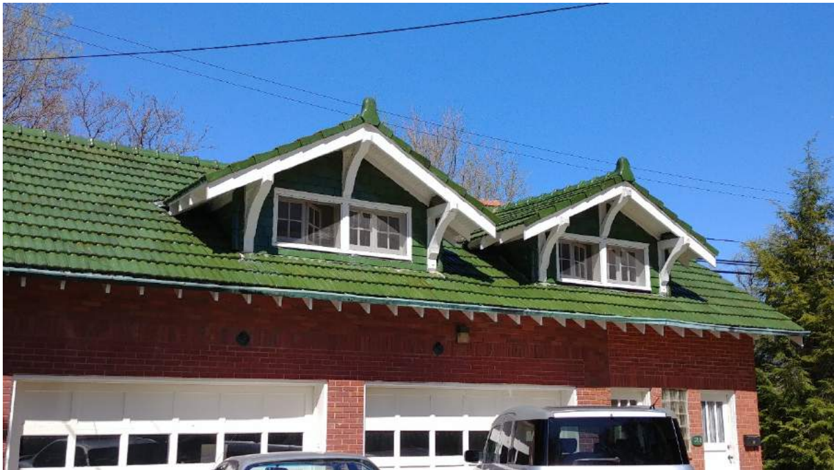
Clay tile roof and dormer detail - Garage
