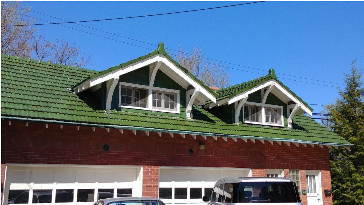
Clay tile roof and dormer detail - Garage
