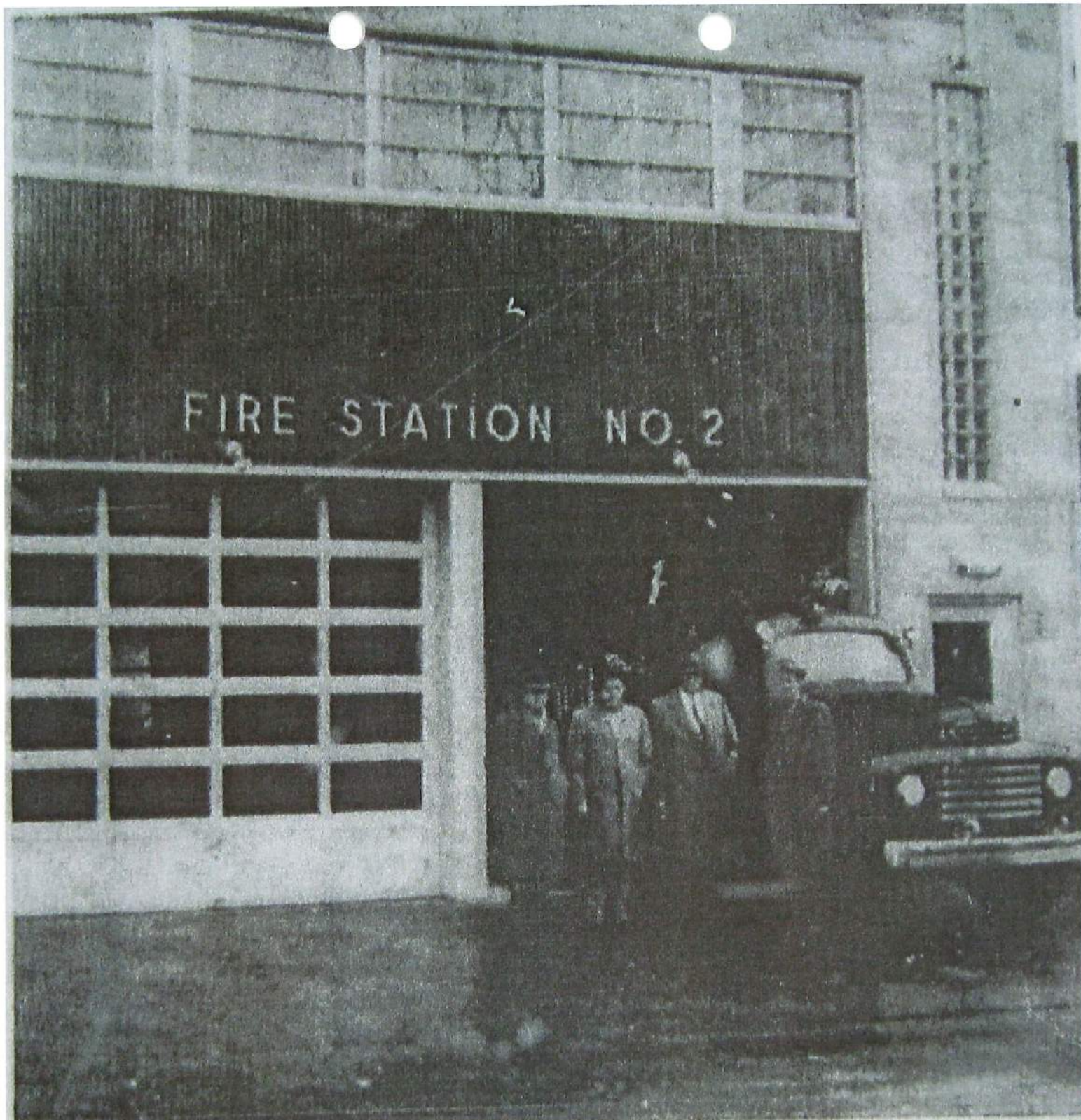
CHRISTMAS GIFT TO CITY —Opening of new $50,000 Fire Department Substation, Kirkwood and Rogers, was announced this week, and operation began today. Shown above are persons instrumental in building station. From left, Architect William J. Strain, Joe Archer, of Upholsters Union, who donated land, Mayor Emmett Kelly and Fire Chief Horace Robertson.
