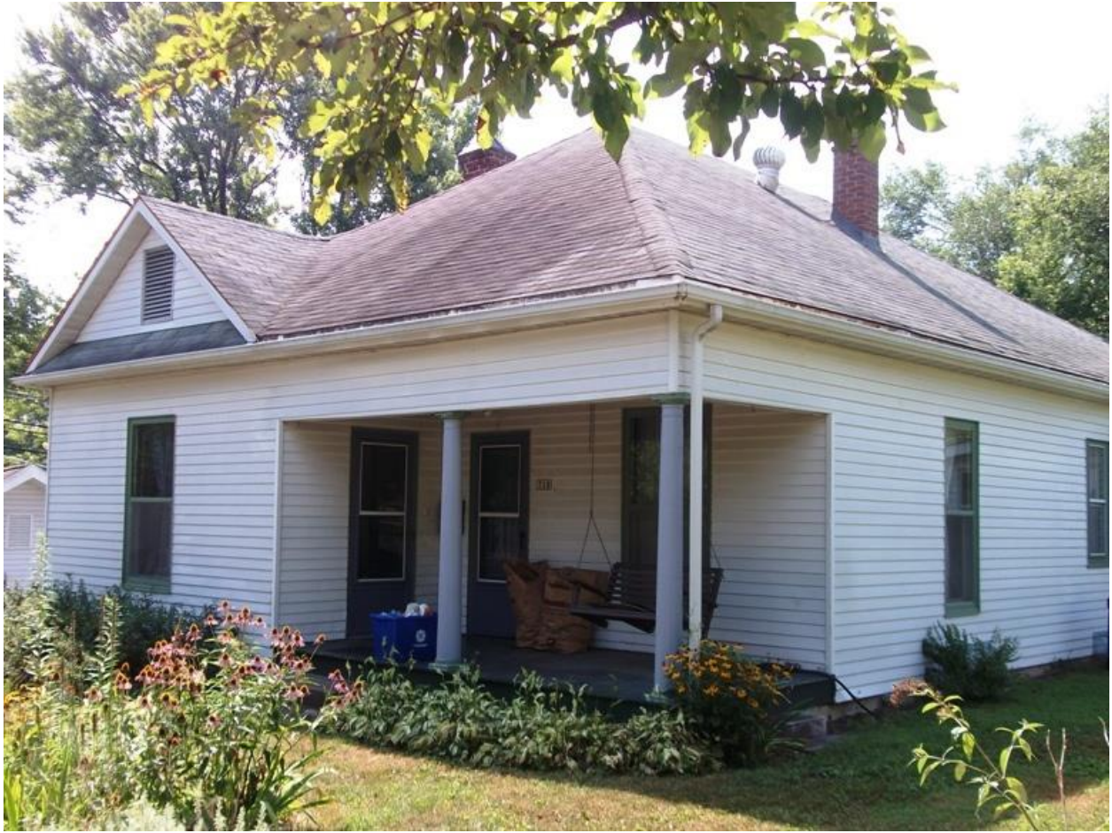
Figure 10. Blair family house constructed by James N. Blair – 715 W. 13 th Street – Contributing
