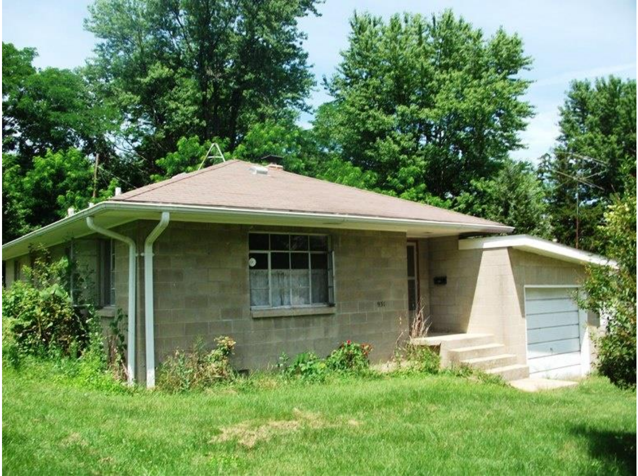
Figure 17. 931 N. Fairview Street – Contributing
