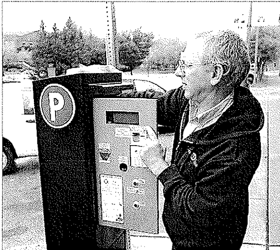
Roy Farris, an employee of EvensTime, installs a new parking pay station on Morton Street in this photo from May 2011. The kiosks accept credit cards or coins and operate in English, Spanish, French and German. David Snodgrass | Herald-Times
