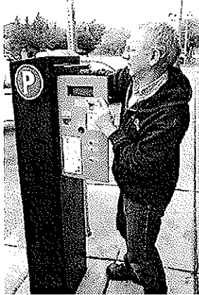
Roy Farris, an employee of EvensTime, installs a new parking pay station on Morton Street in May 2011. The pay stations replaced parking meters, accept credit cards or coins and operate in several languages. The use of similar stations is being proposed for much of downtown Bloomington's on-street parking. David Snodgrass | Herald-Times
