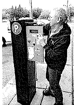
Roy Farris, an employee of EvensTime, installs a parking pay station last year on Morton Street. The kiosks replaced parking meters near Bloomington's City Hall. They accept credit cards or coins and operate in several languages. Similar pay stations are being discussed for downtown streets. David Snodgrass | Herald-Times
