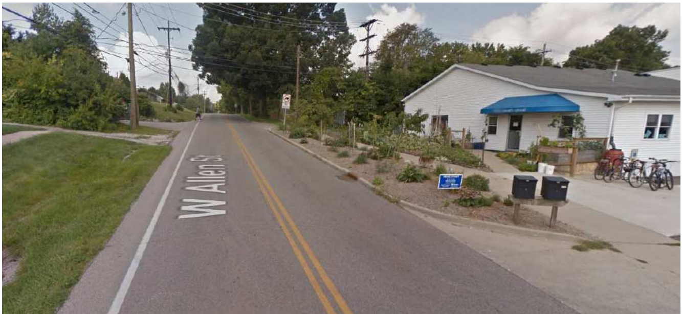
Figure 2: Looking west between Strong Drive and Larkspur Lane (Google data 2014)
