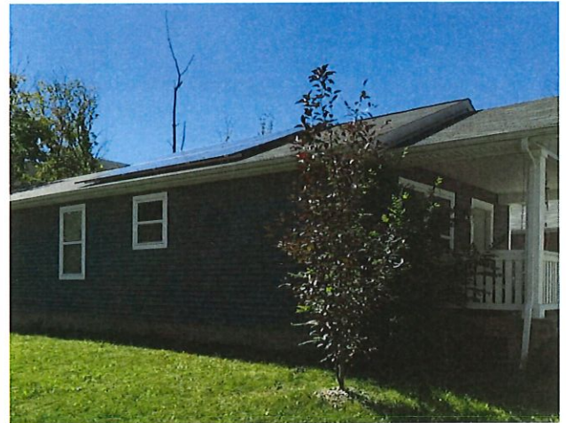
Installation of proposed solar panels on similar house.
