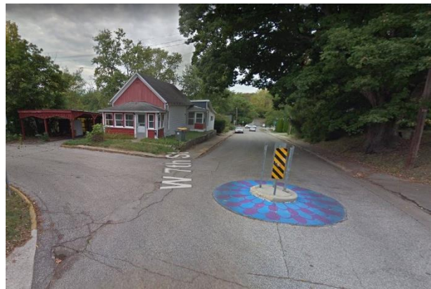
Traffic circle on West 7th Street (Bloomington, Indiana)
