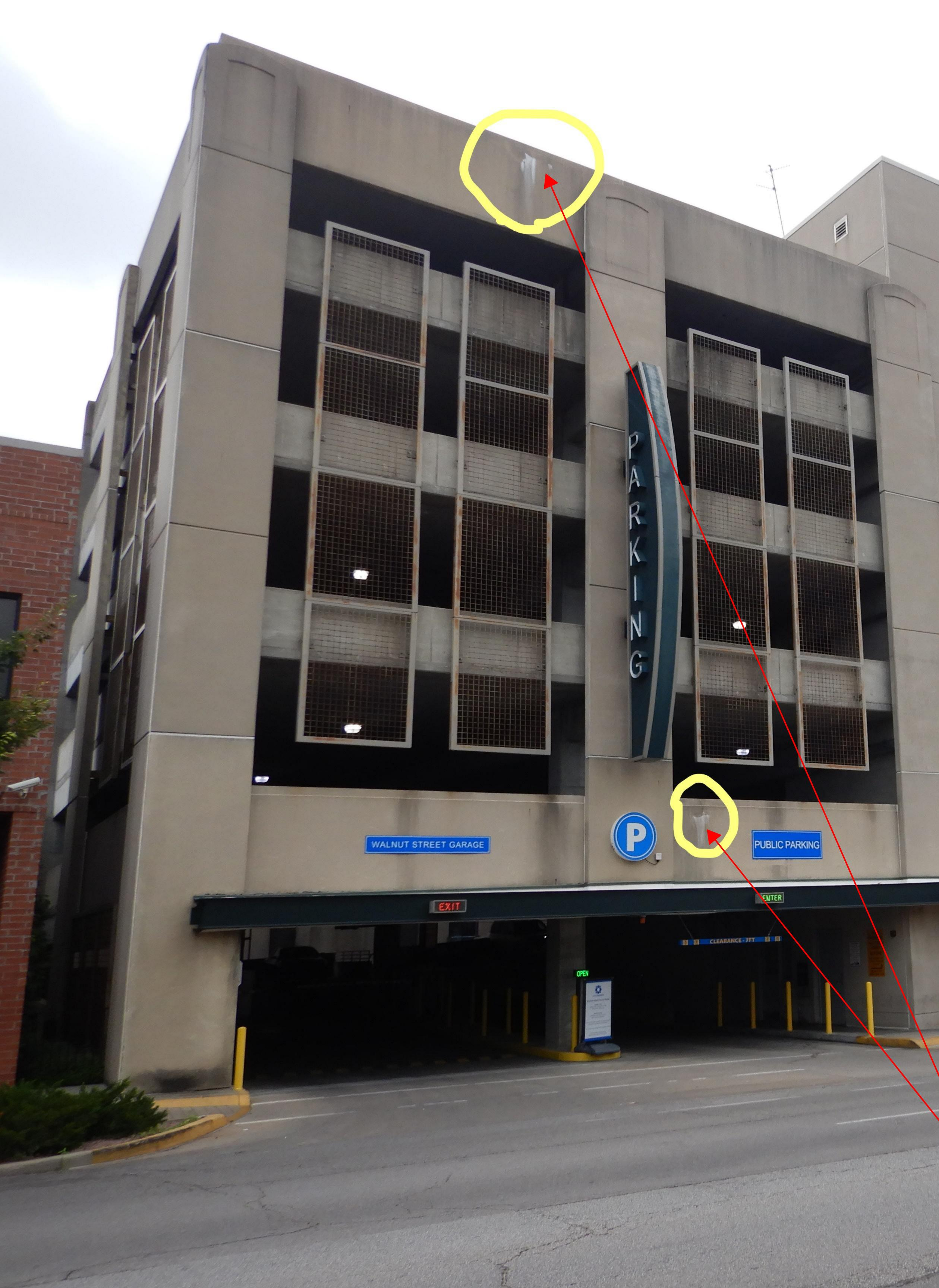
URGENT REPAIR: AT TWO LOCATIONS NOTED, ADEQUATELY PROTECT SURROUNDING AREAS FROM DAMAGE, INCLUDING SIDEWALK BELOW, AND REMOVE ALL LOOSE CONCRETE. IF REINFORCING STEEL IS EXPOSED, COAT REBAR WITH ANTICORROSION AGENT AND ALLOW TO CURE.
